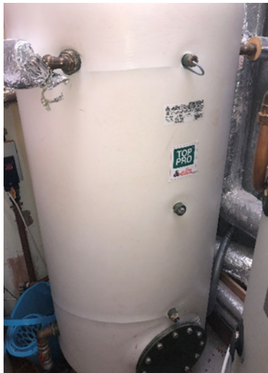
Figure 51 Naíolann Árann Childcare Facility plant room. Left: existing buffer storage tank (300 L approx.), and right: existing 310 L DHW cylinder with internal heat exchanger coils.
