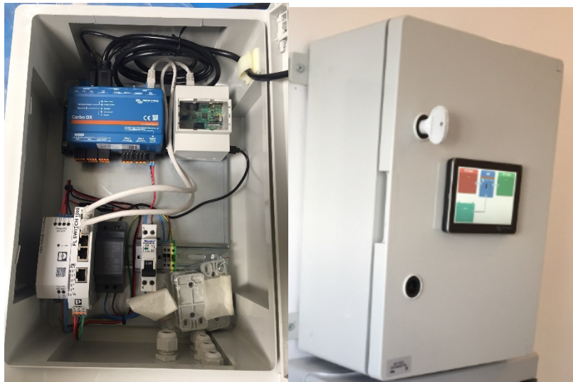
Figure 19 Monitorization cabinet
