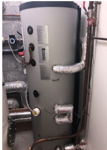
Figure 51 Naíolann Árann Childcare Facility plant room. Left: existing buffer storage tank (300 L approx.), and right: existing 310 L DHW cylinder with internal heat exchanger coils.
