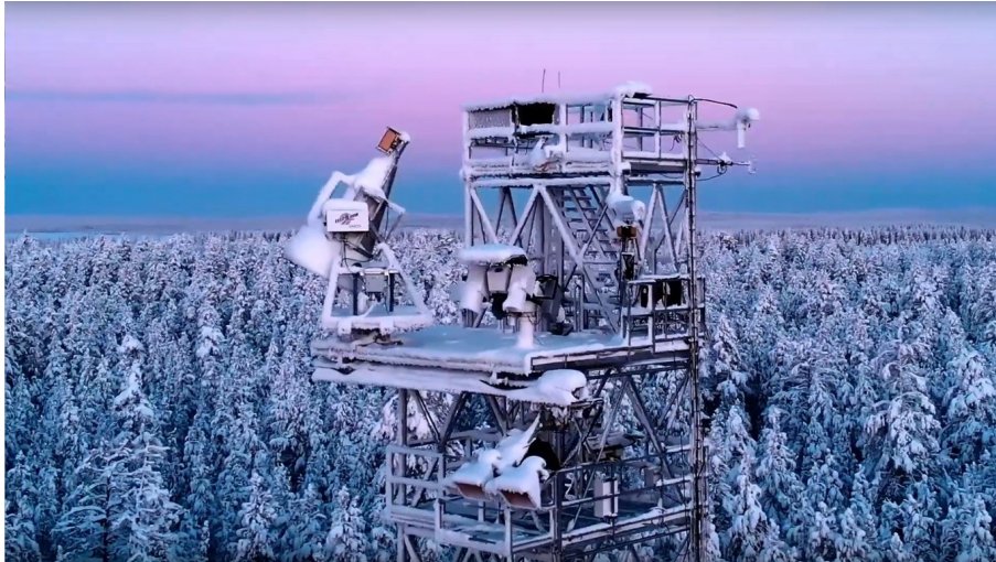
Figure 16: Microwave instrumentation installed on the top platform of the ICOS tower at FMI-ARC. SodScat is lowermost, attached on a rail at the base of the platform.
