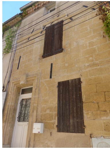
(b) Stone masonry with tie rods to link floors with the facade (Rue de l'église, Rognes).
