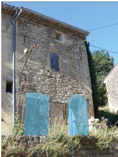
(a) Filling of two openings (in blue) close to the building corners (Rue de l'église, Rognes)
