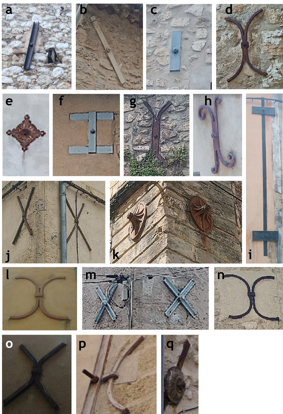
Figure 19: Typology of tie rods used in Lambesc (e, f, g, h, j, k, o), Saint-Cannat (a, b, c, d, l, m, n) and Rognes (i, p, q)
