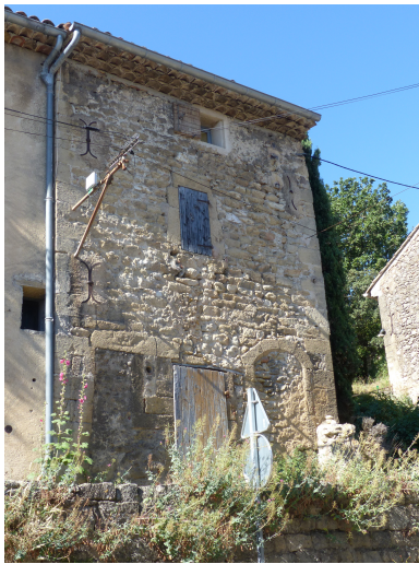
(a) Stone masonry with tie rods to link floors with the facade (Avenue de Lambesc, Rognes).
