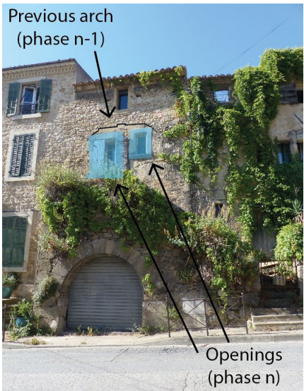
(b) Filling of a previous arch and arrangement of two openings
