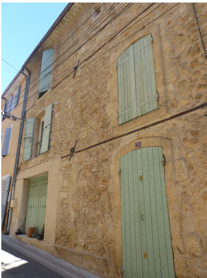
Figure 22: Reconstruction along the window (first floor). Metal tie rods.
