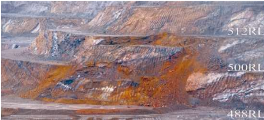
Fig. 7. Pit slope failure propagation to 15 m high contained within a larger failure catchment bund on 26 November 2019–pit floor 488 RL.
