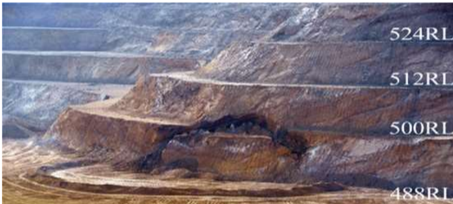
Fig. 6. Pit slope with initial 8 m high failure contained within a rock fall catchment bund on 26 October 2019–pit floor 492 RL
