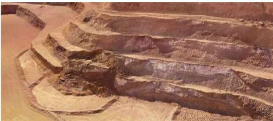
Fig. 10. 3D model developed from UAV photogrammetry with the planar failure on the left hand side near the convex slope profile. Lighter colored material on the right hand side where repetitive bench crest losses have occurred shows near-planar shale bedding planes. Shape accuracy is <math><5\text{ cm}</math> without GCP.
