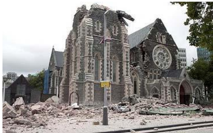
Figure 7: Christchurch Cathedral after the Earthquakes in 2011 (Telegraph 2011)
