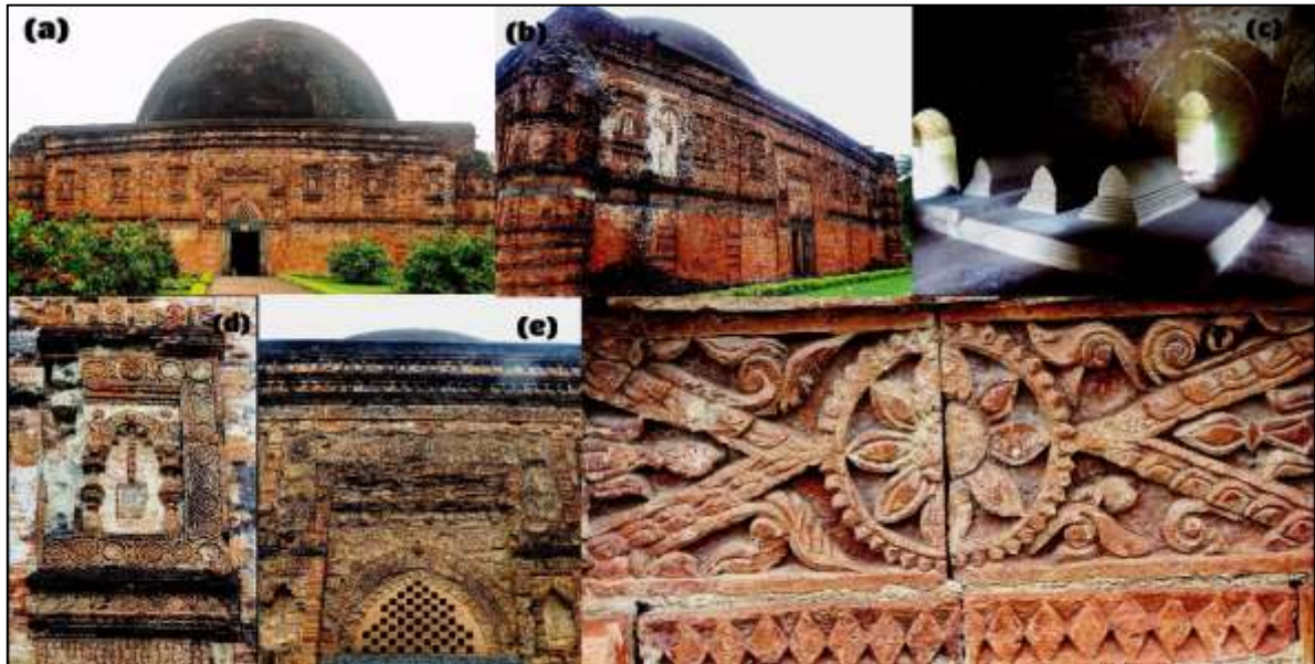
Figure 10. (a) Frontal view along with stone doorway of Eklakhi Mausoleum, (b) Octagonal turret, (c) graves are of Jalaluddin and his wife and child, (d) & (e) Terracotta ornamentation along with floral panels on the exterior walls, (f) Details of terracotta work in the panel.
