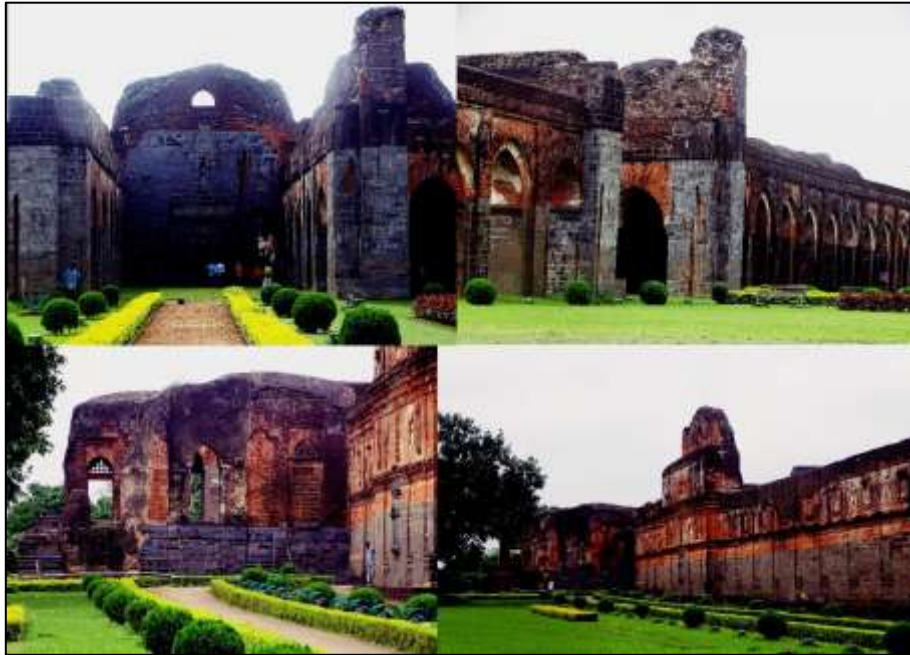
Figure 11. Exterior view of Adina Mosque
