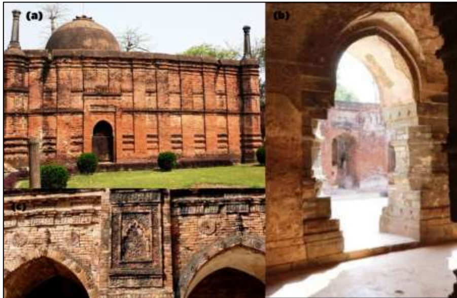
Figure 6. (a) Front view of Kadam Rasul Mosque showing the marble towers on the corners, (b) One of the arched openings, (c) Ornamented exterior wall of the mosque.
