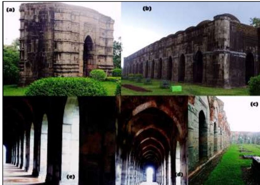
Figure 2. Different portions of Baro Shona Mosque (a) Courtyard gateway, (b) Exterior part, (c) External (interior) wall of the ruined musalla with marks of fallen domes, (d) Arched pattern of the interior portion, (e) Aisle.
