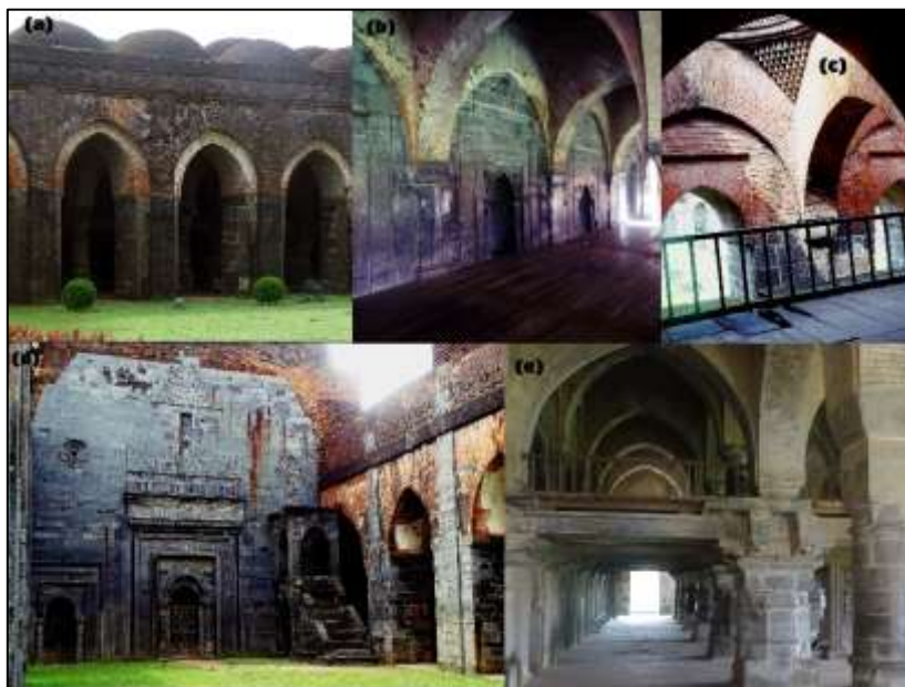
Figure 12. Different Architectural parts of Adina Mosque. (a) Small domes raised over each bay supported by pendentives. These pendentives were formed of brick built in oversailing courses, (b) Mihrabs, (c) Range of arches carried by pillars, (d) Central nave of the sanctuary is in the form of a well-proportioned hall aligned east and west earlier had a barrel vault, (e) Pillars of prayer hall which are Graceful fluted shafts and carried different arches.
