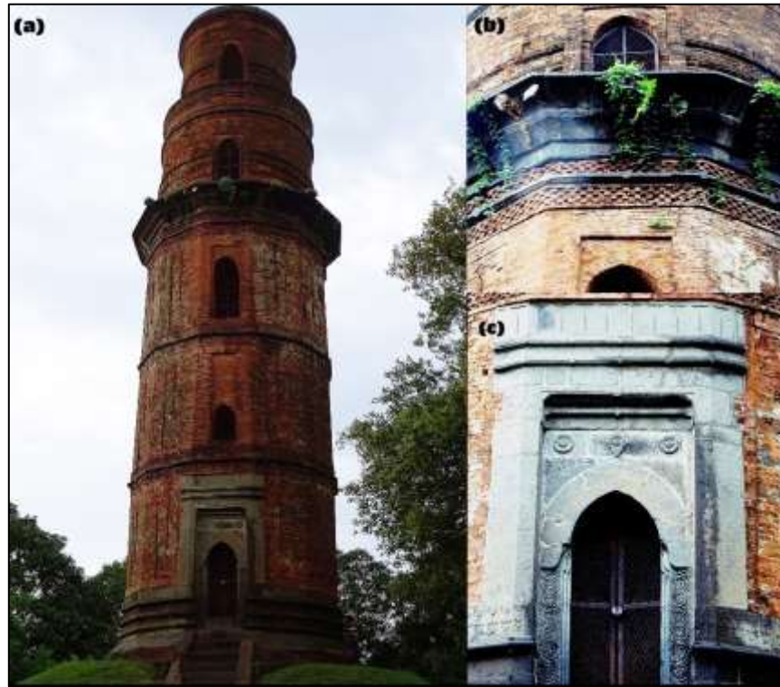
Figure 4. (a) Firuz Minar/ Firoz Minar, (b) Terracotta curving on the outer wall, (c) Granite made entrance.
