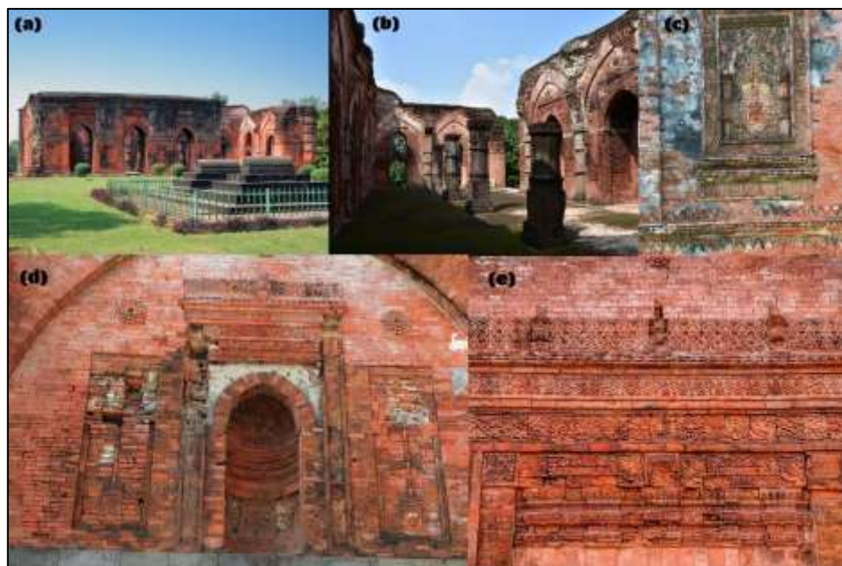
Figure 9. (a) Frontal view of Tantipara Mosque, (b) Inside of Tantipara Mosque with marks of fallen domes, (c) Terracotta floral panel stands out in the high relief against the plain wall (exterior), (d) & (e) Rich terracotta ornamentation.
