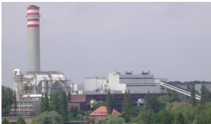
Fig.6.View of EPS Pomorzany, Szczecin. Flue gas humidifier tower of EBFGT plant – front left.
