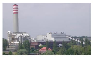
Fig.6.View of EPS Pomorzany, Szczecin. Flue gas humidifier tower of EBFGT plant - front left.
