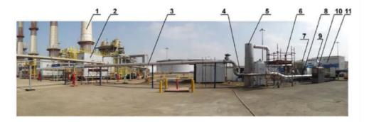
Fig.11c General view of the pilot plant at the Jiddah Refinery. (1) stack of boiler, (2) boiler, (3) flue gas duct, (4) pilot plant control room, (5) gas conditioning column, (6) pilot plant stack, (7) cartridge bag filter, (8) thermal insulated duct, (9) cyclone, (10) ammonia dosing unit, (11) mobile accelerator unit.
