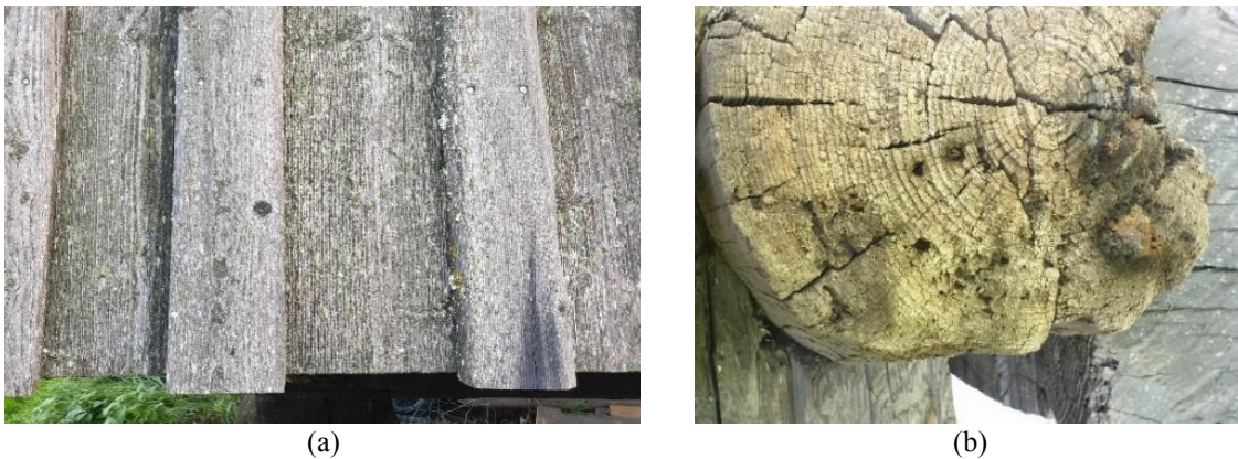
Figure 7: (a) Lichen attack to the coating, (b) Insect attack on the timber logs
