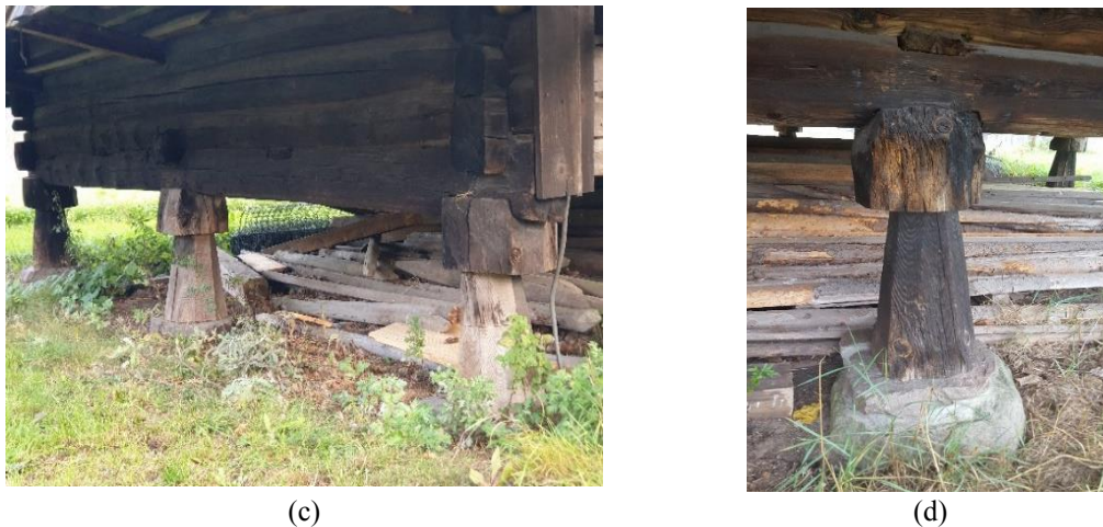
Figure 6: (a) Fadum Storehouse view, (b) Structural detail inside the coating, (c) Timber short columns under the building, (d) detail of the simply connected timber column
