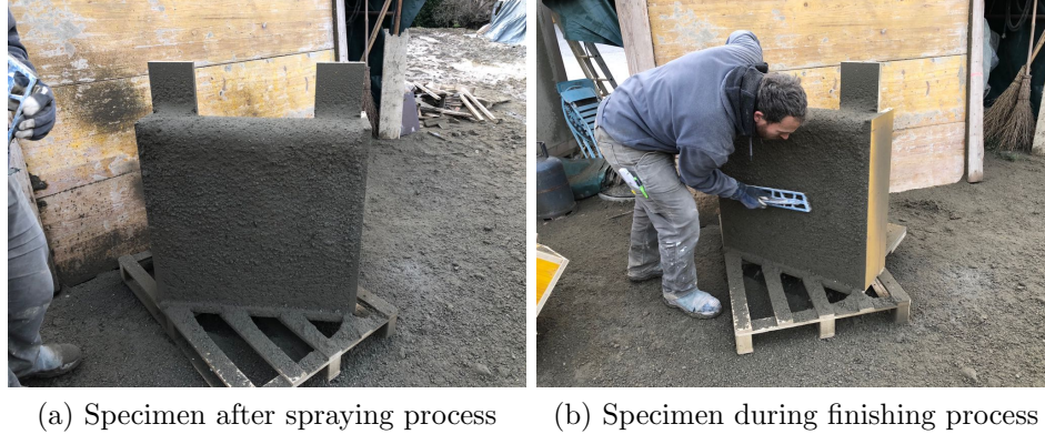
Figure 4: shot-earth spraying technology
