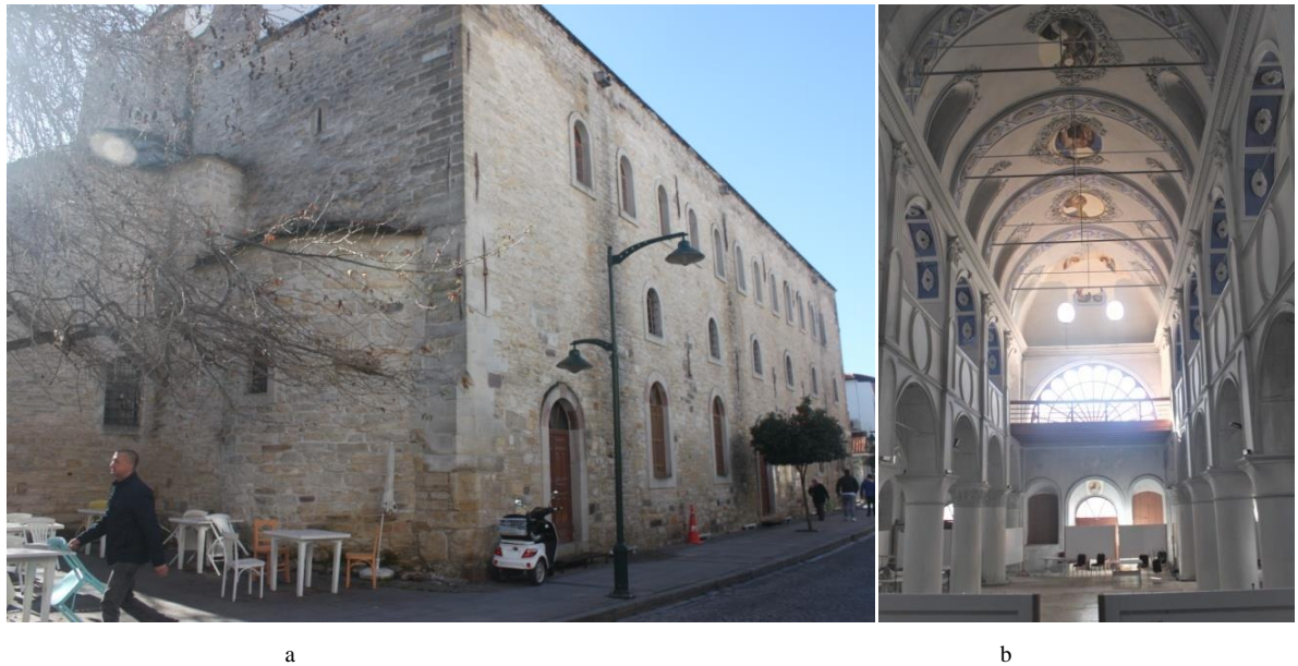
Figure 7. St. Haralambos Church after the restoration; (a) east facade, (b) interior view (Severoğlu, 2019)
