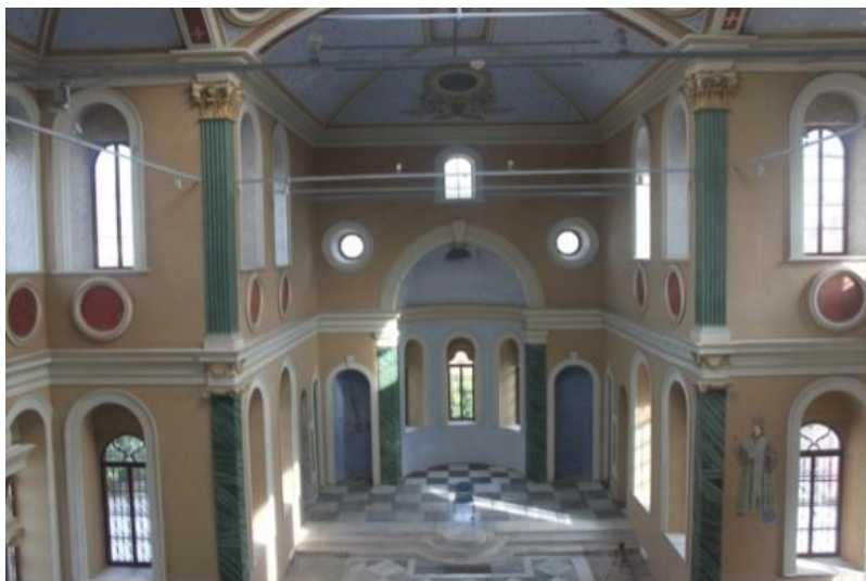
Figure 5. Interior view of the church after the restoration (Severoğlu, 2018)
