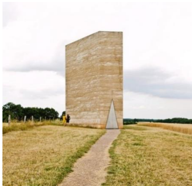
Figure 15. Bruder Klaus Field Chapel. (Source: https://www.archdaily.com/106352/bruder-klaus-field-chapel-peter-zumthor )
