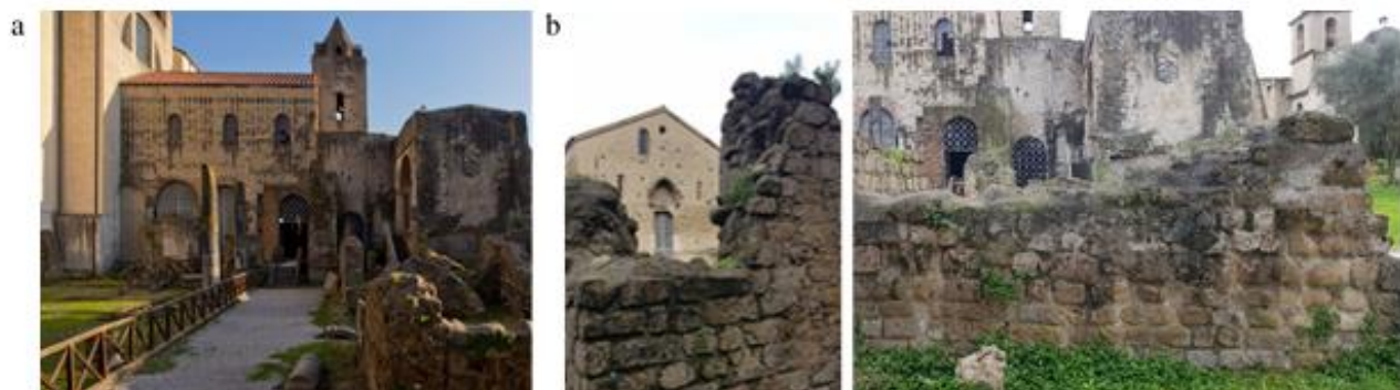
Figure 1. (a) Complex Paleocristian Cimitile: Basilica nova; (b) Details of protection of crests of walls with a technique called "spalmata" of mortar
