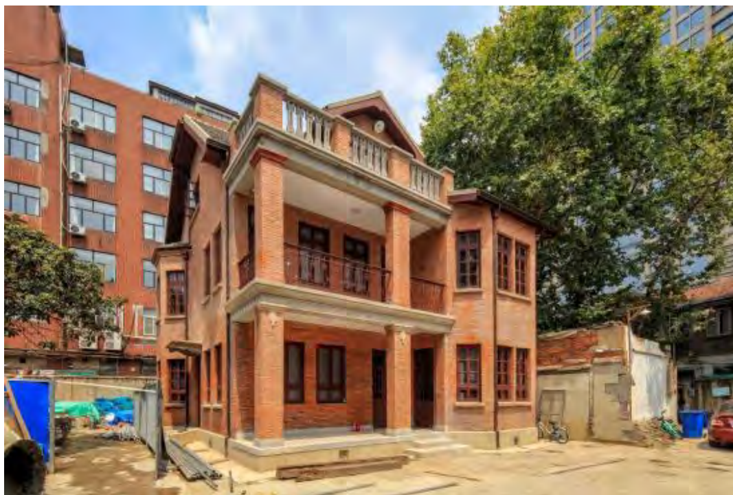
Figure 25 Building No.2 after conservation (Image source: photographed by the author)
