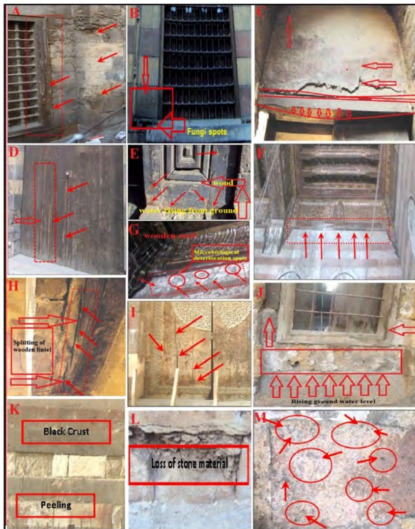
Figure 2. Deterioration features of limestone and wooden elements of a case studies : A-Loss of stone material and separation of wood texture, (Al maridani mosque), B-Fungi spots on limestone's surface (Madrasa of Qanibay alammah), C- Deflection of wooden lintel due to fissures in wall, D-Cracking and flaking of paint layer of wooden door (Madrasa of Sultan Hassan), E-Flaking and crumbling of paint layer, F-Separation of wooden roof from wall (AlMahmoudia Mosque), G- Black spots on limestone surface, H- Splitting in the wooden lintel, I-Splitting in wooden door and the paint flakes with thick layers dropping off (Madrasa of Gawharal-Lala), J-Loss of stone material, and separation of wooden texture , K-Black crust and peeling , L-Loss of stone material, M- Pitting in limestone surface.
