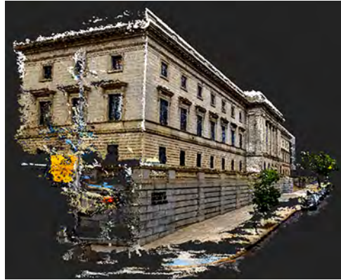
Figure 7. PHOTOGRAMMETRY It is a series of overlapping images taken for the object and then several possibilities exist for the outputs, including ortho-images, and textured meshes. (photogrammetry — photography & architectural photogrammetry, 2019)
