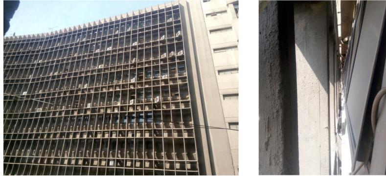
Figure 2. Building Façade view from Windsor Hotel (Left) and the Deteriorating Façade System (Right) \*Photos taken by Co-author
