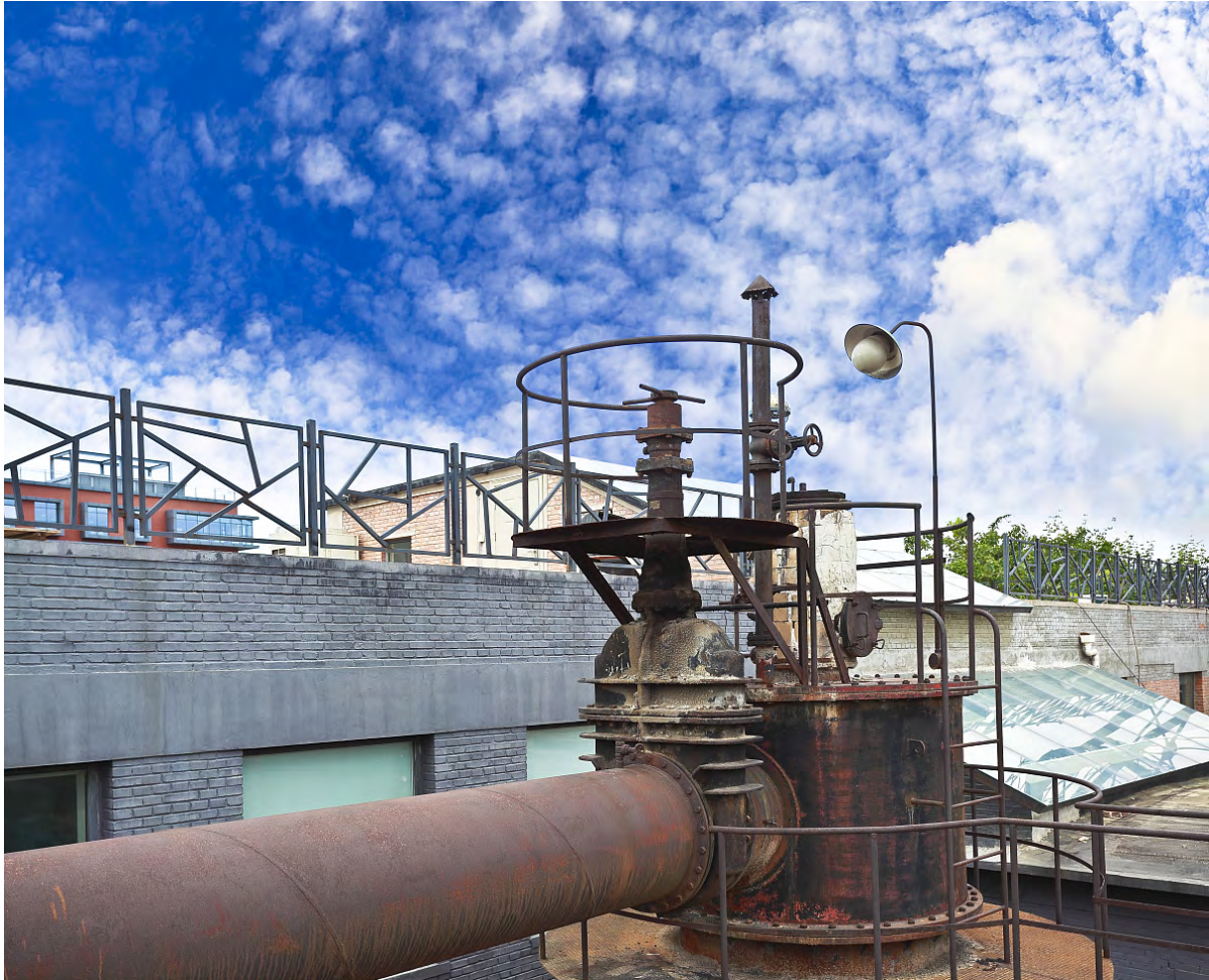
Figure 1. Abandoned factory in the city (Source: www.quanjing.com )
