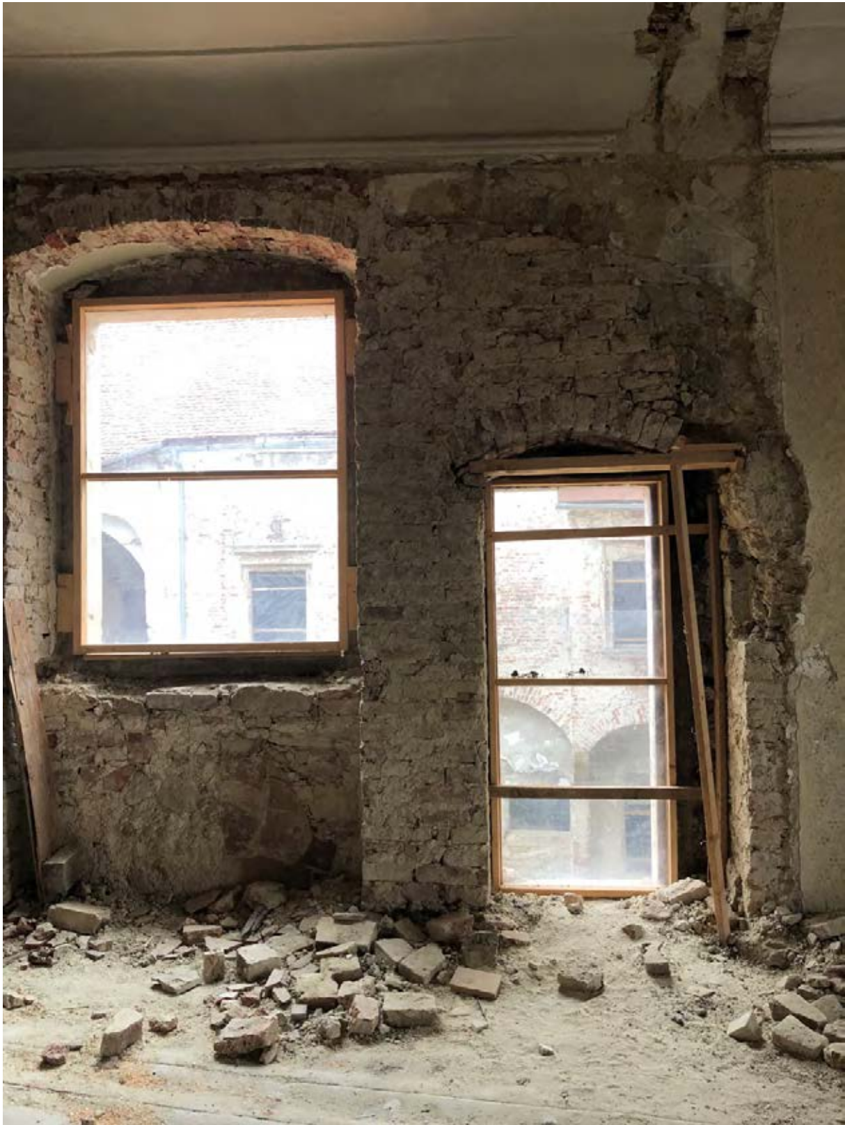
Figure 17. Man-made cause, destructive research method, recent opening of historic doors and windows
