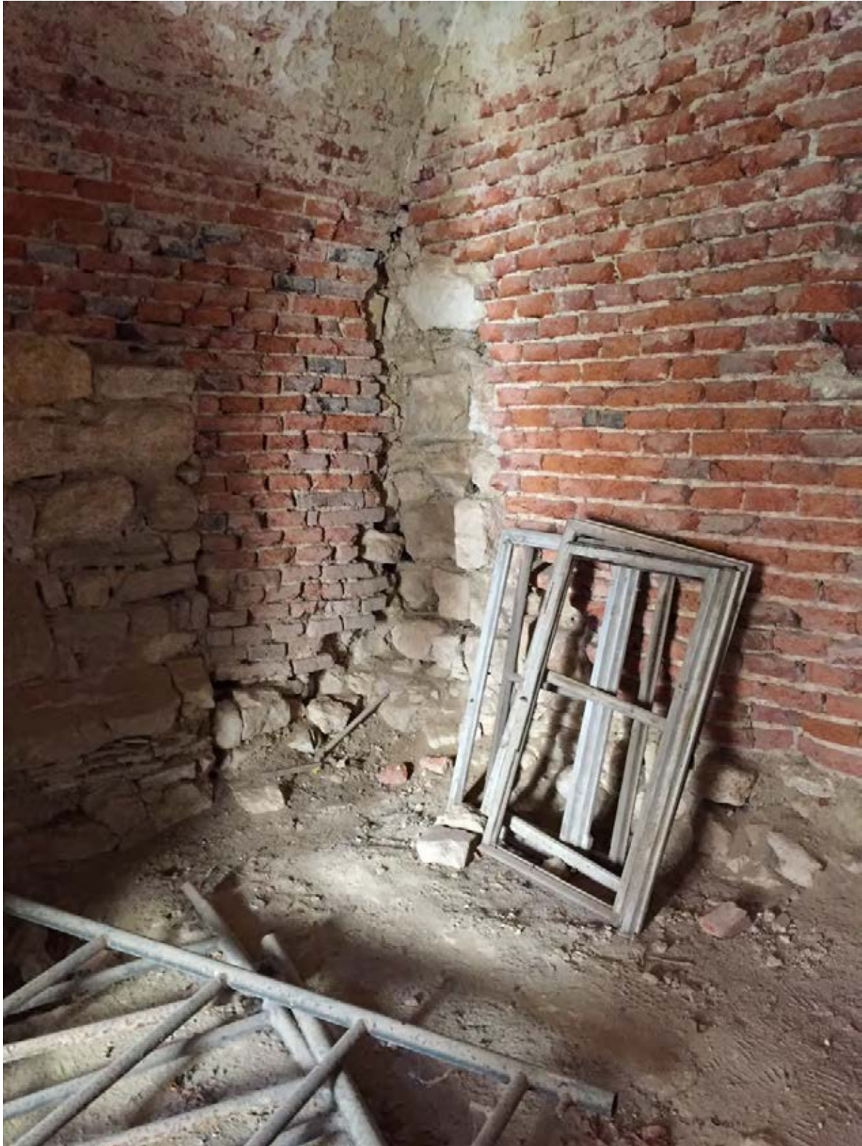
Figure 8. Remains of the original supporting wall
