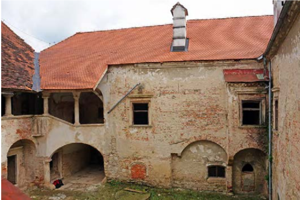
Figure 6. Courtyard, south-east wing
