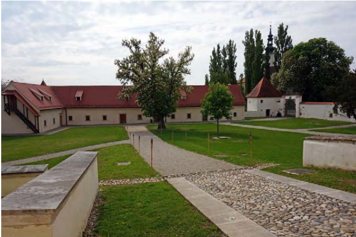
Figure 23. View on the rebuild part of Castle Complex
