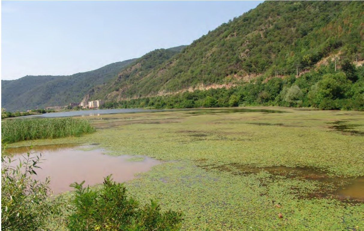
Fig. 64 Cozla pond, formed behind a dam part of the mining facilities
