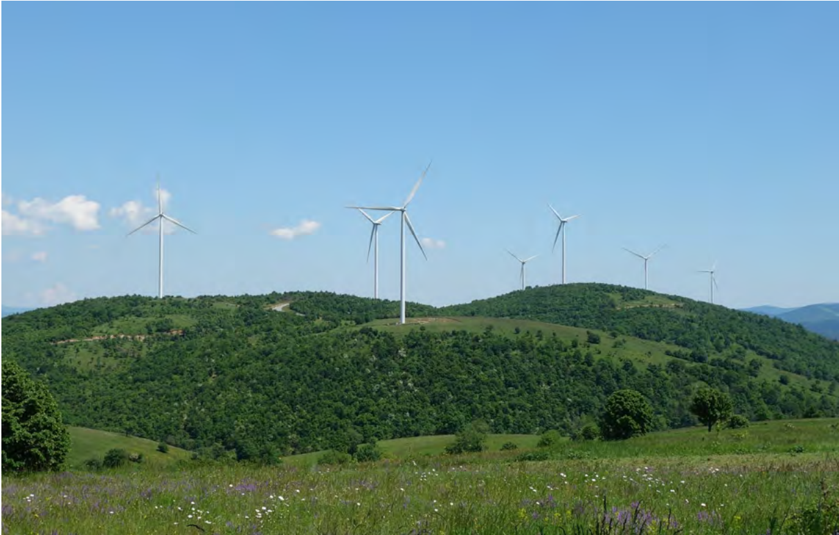
Fig. 65 Sfânta Elena Wind Farm constructed near Coronini town
