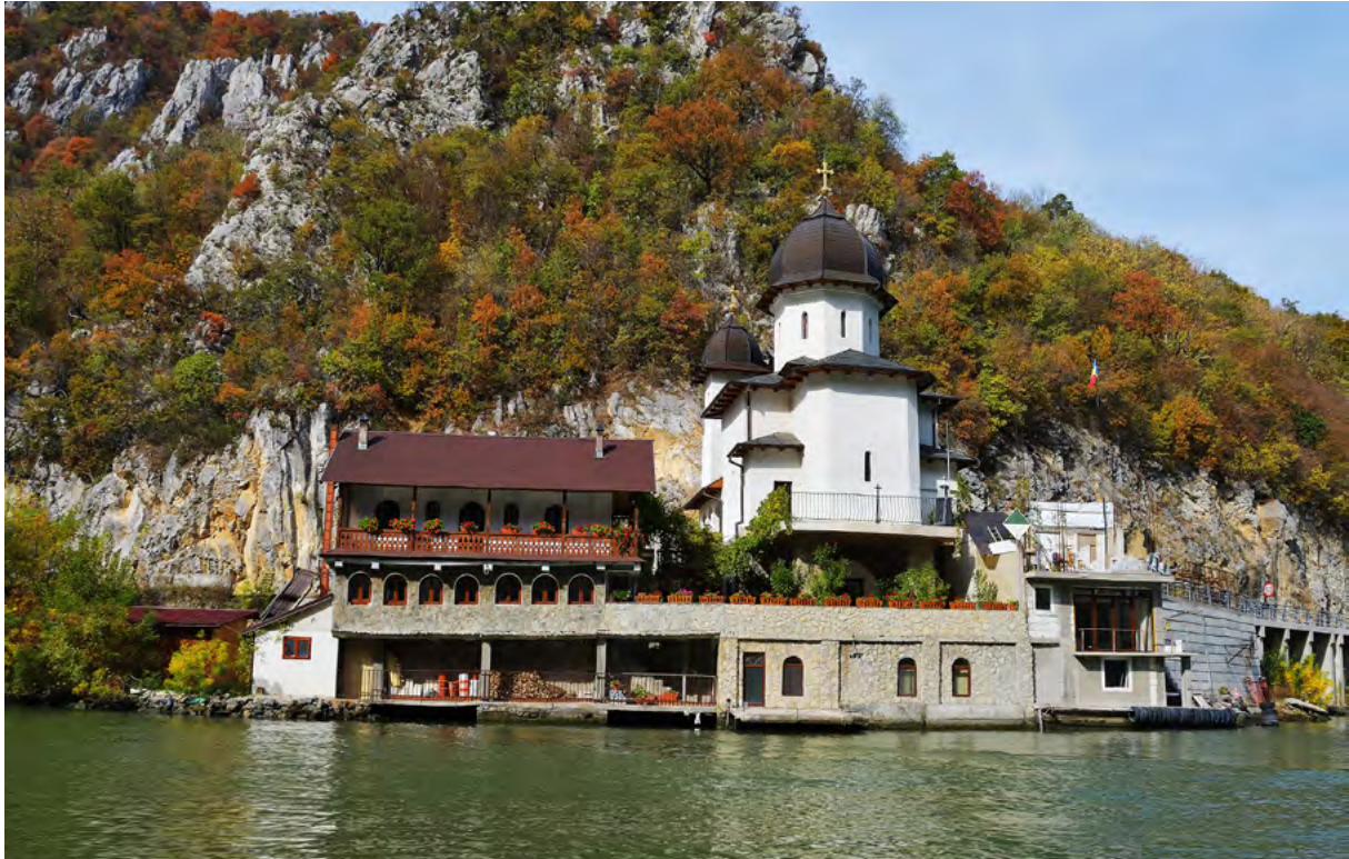
Fig. 68 The Mraconia Monastery was constructed on a former observation point of the Danube navigation
