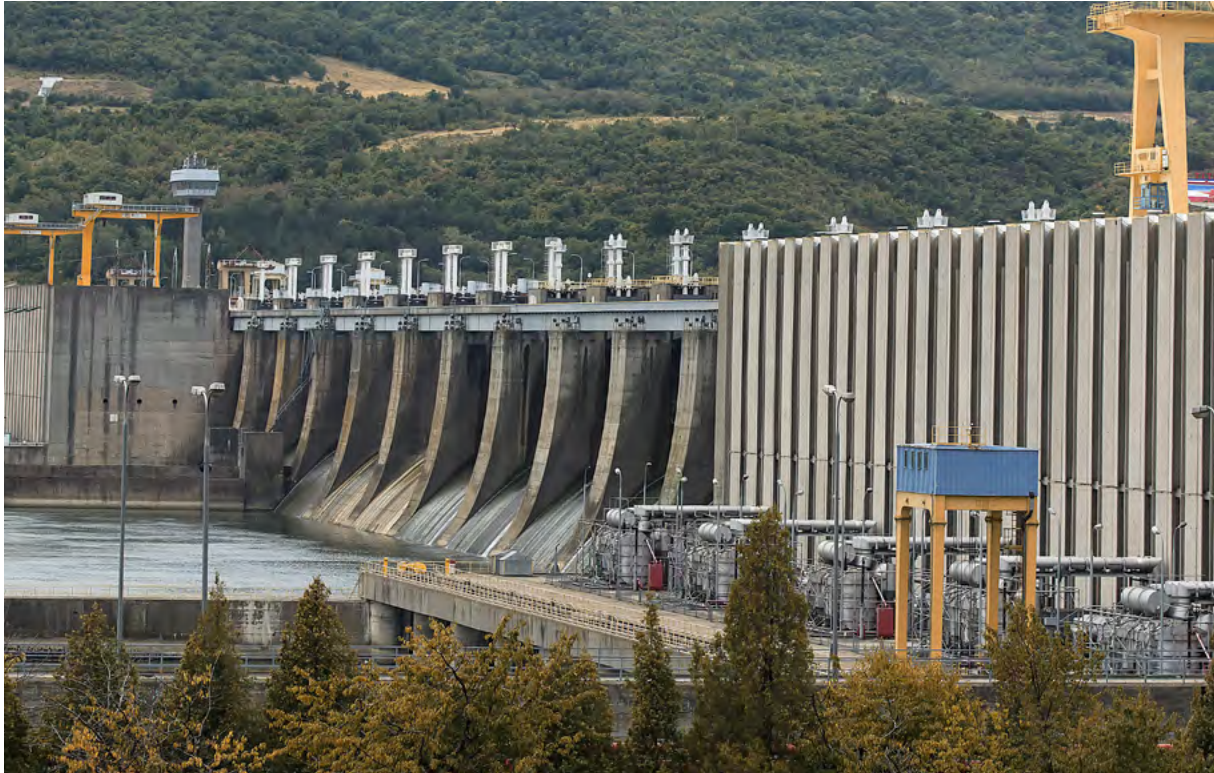
Fig. 11 Iron Gates I Dam, located at km 943 of Danube River. Its construction changed the flowing regime of Danube upstream, from river to lake-like (reservoir). This lake-like regime is evident up to Belgrade (Serbia)
