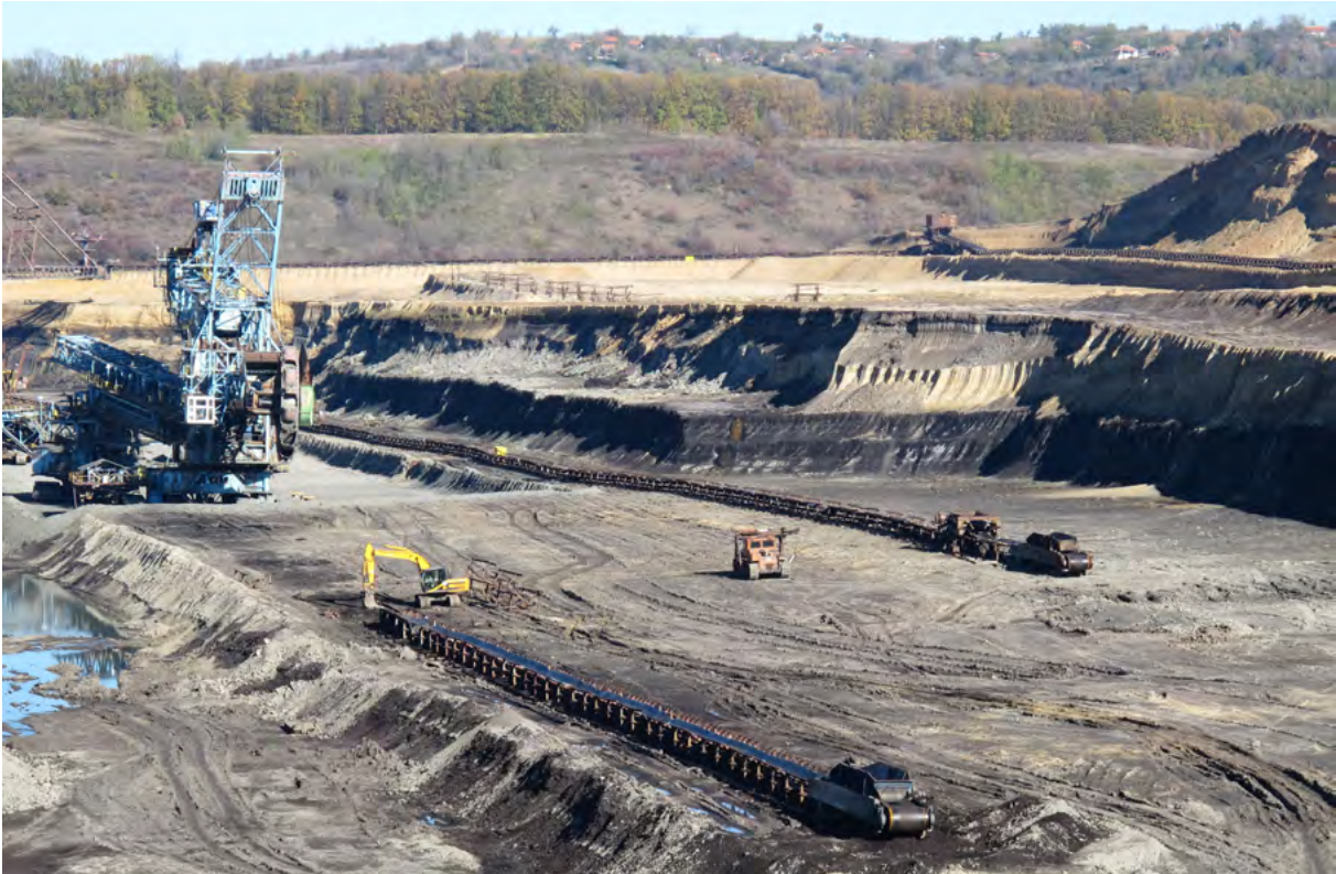
Fig. 51 Husnicioara open cast mine, close to Drobeta-Turnu Severin, for Pliocene (Dacian – Romanian) lignite, Dacian Basin
