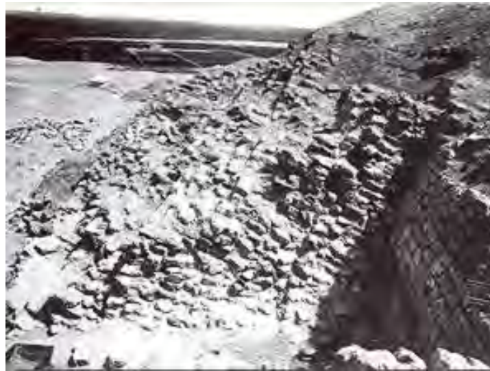
Figure 2. Part of the unfinished pyramid at Saqqara. Mud bricks as a building material were handy to transport on ramps then piled in inclined to 75^{\circ} walls.
