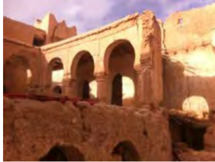
Figure 4. Example of a deteriorated house of Moussani
