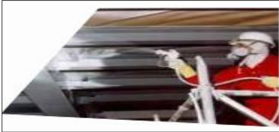
Fig. 5: Intumescent coating spraying procedure
