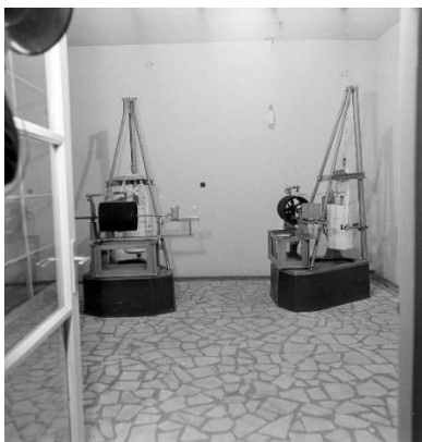
Figure 7 – Mainka Modified seismographs with 540 kg mass (left) and Mainka seismographs with 180 kg mass (right) at the Timișoara seismic station (Source: Timișoara seismic station Archive).
