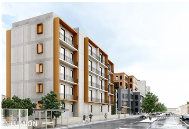
Figure 19: Coplanar ceramic tiles that are all bound together through a rigid substructure.
