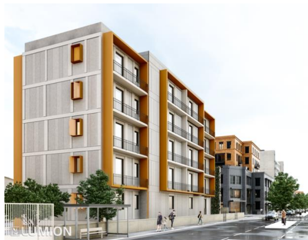
Figure 20: non-coplanar ceramic tiles that are all bound together through a rigid substructure. This expedient emphasizes the compositional rhythm of the e-SAFE panels and the geometry of the stringcourses.
