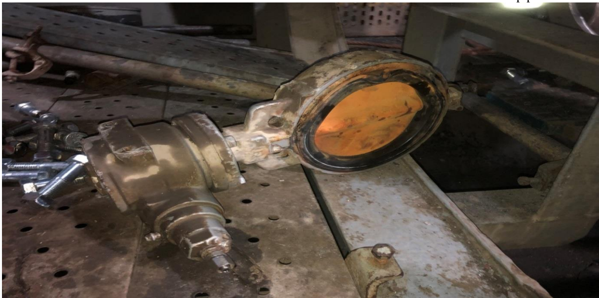
Photo 5. Cargo flap (during repair)
