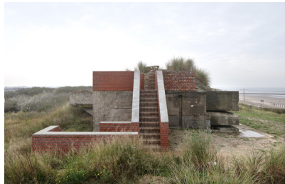
Image 19: addition in bricks bunker n°1, credit Filip Dujardin 2021.
