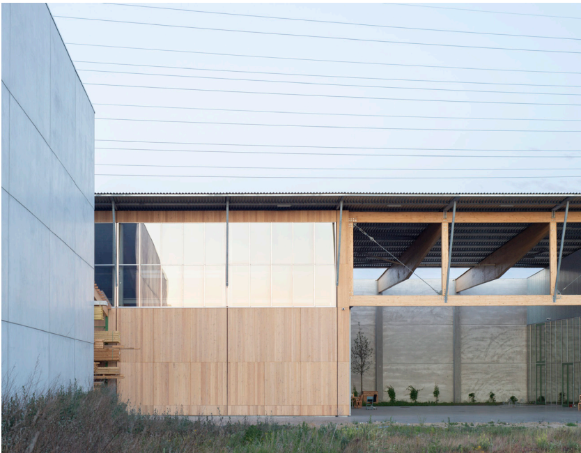
G1812 Industrial building, Gent (BE), 2021, GAFPA. A facade of prefab wooden panels mirrors the concrete replica's of the neighbours.
