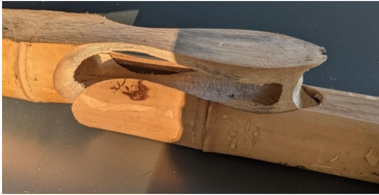
a) CNC routed splice joint
