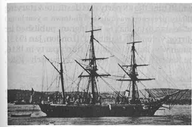
HM screw sloop Falcon at anchor in Sydney Harbour 1867. She formed part of the RN squadron on the Australia Station from May 1864 to October 1867. With her funnel housed (folded down) she has the appearance of a sailing ship (barque rig).
