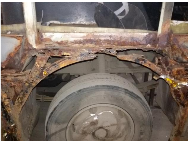
Fig. 3. Destruction of the frame of the bus body under the influence of corrosion
