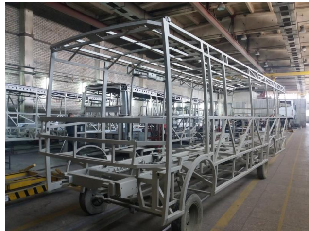
Fig. 4. The body frame of the bus, which is covered with high-adhesion anticorrosive primer
