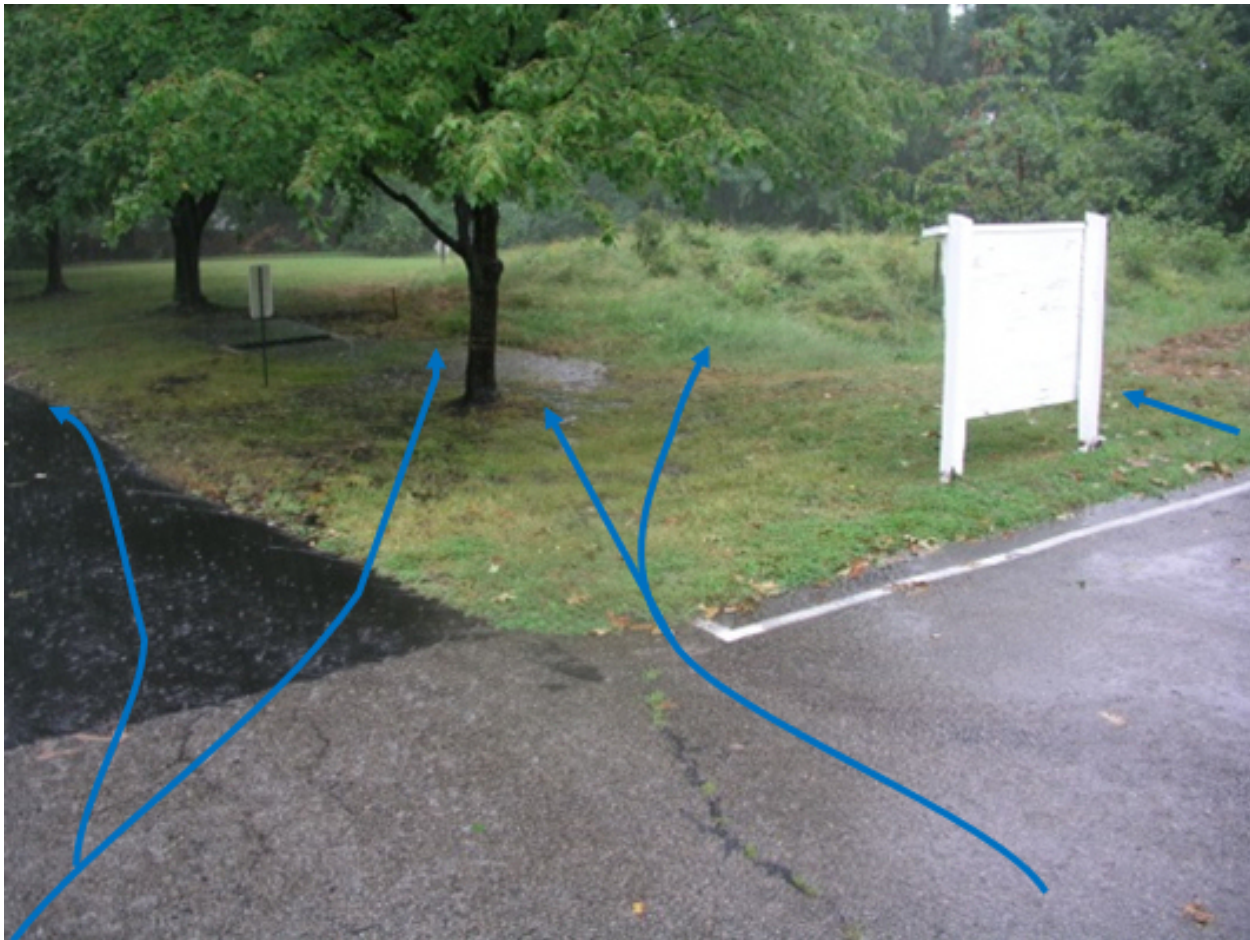
Figure 2-15. Multiple input pathways for rain garden
