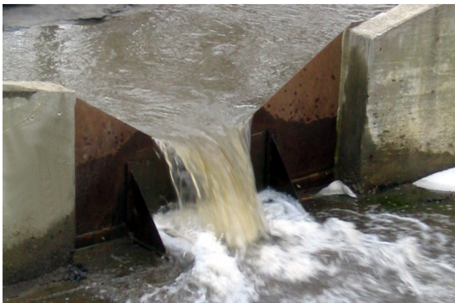
Figure 3-3. 120° V-notch weir, Englesby Brook, Burlington, VT
