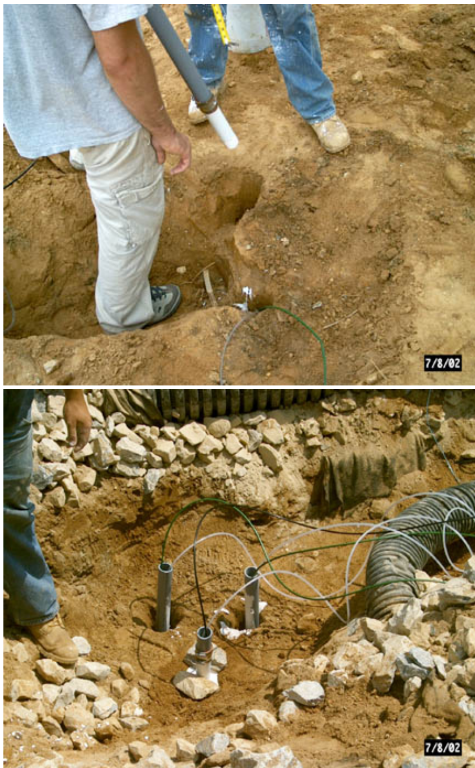
Figure 3-40. Lysimeters before and after installation (photos by R. Traver, Villanova University)
