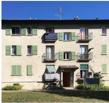
Type 4 : Continuous balconies
