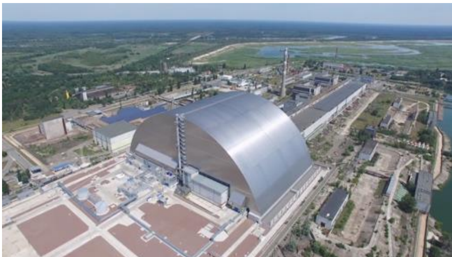
New Safe Confinement (NSC or Arch) was moved over the Shelter Object in November 2016. Complex NSC-SO
