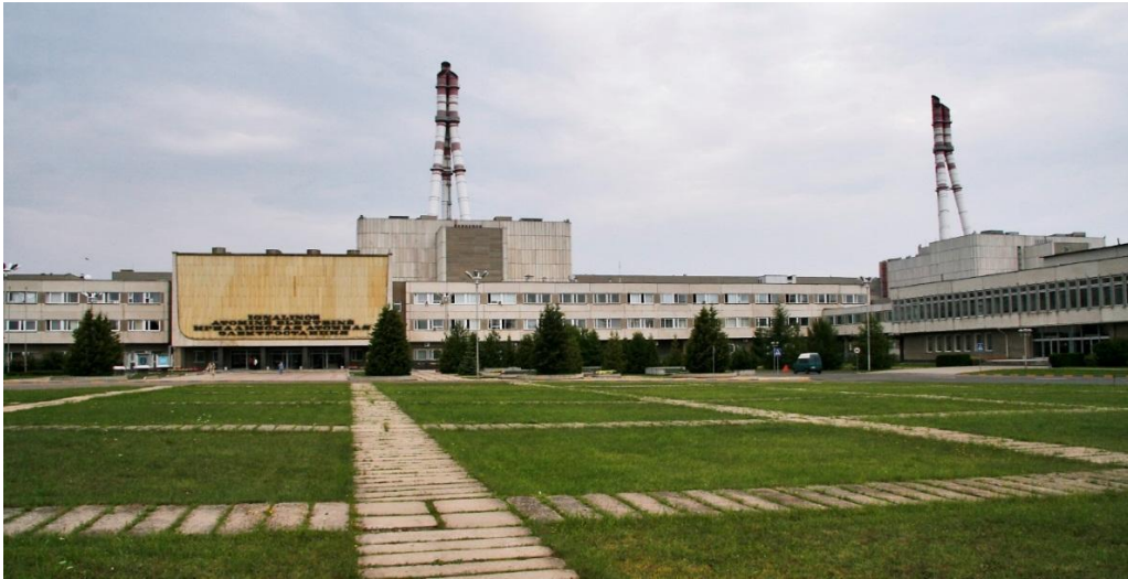
Ignalina Nuclear Power Plant Lithuania with two towers
