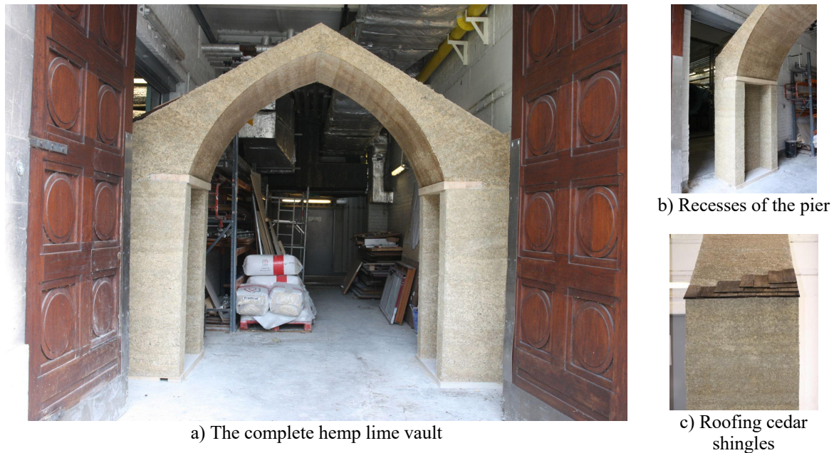
Figure 2: The hemp lime vault built during the Vertical Studio 2009
