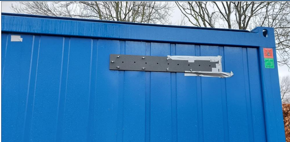
Figure 33 Photo of ventilation opening in the container with a slot with 9 holes.
