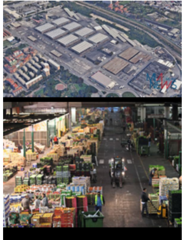
Figure 14: SogeMi Wholesale Market (Source: Polifactory)
