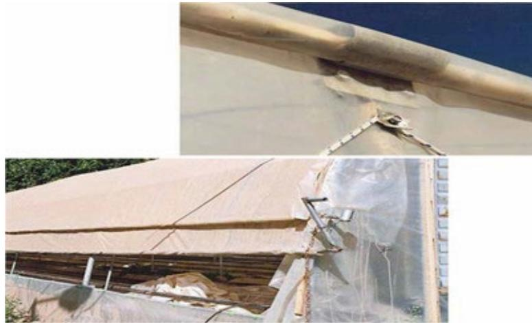
**Figure 3.16** Fixing and stretching both the plastic film of the roof and the ventilation opening on one tube
