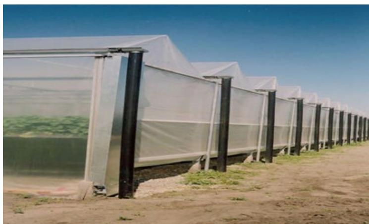
**Figure 3.5 Plastic film cladding, used in mild climates**
