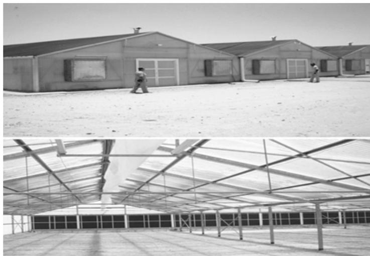
**Figure 3.22** A greenhouse structure for desert regions in Kuwait, covered with rigid plastic sheets and equipped with fan and pad cooling
