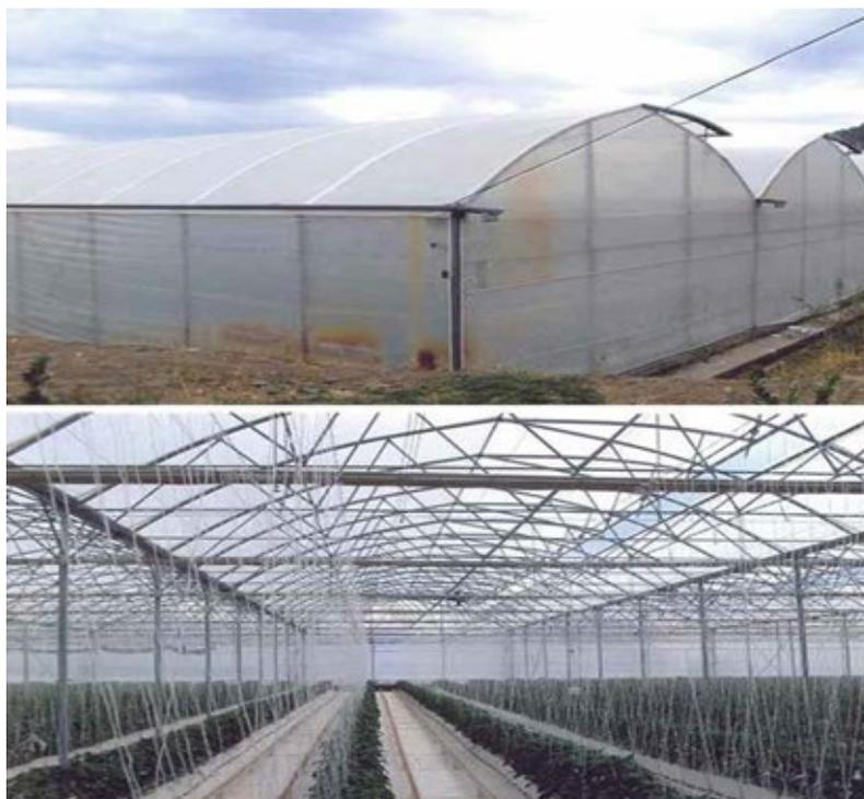
**Figure 3.18 Multi-span greenhouse with flap ventilation at the ridge and roll-up ventilation at the sidewall**
