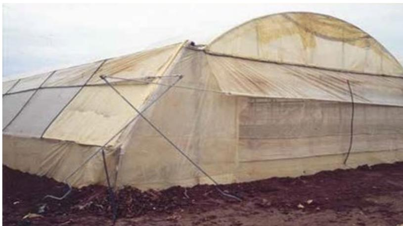
**Figure 3.15 Sloped sidewalls covered with insect screens and rolling-up ventilation**
