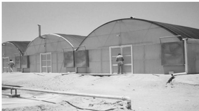
**Figure 3.23** A round-arched structure covered with plastic film and permanent shading net, ventilated and cooled by fan and pad system
