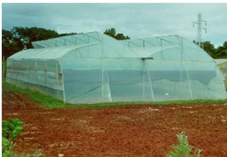
**Figure 3.8 More advanced plastic-covered greenhouse with roof ventilation**
