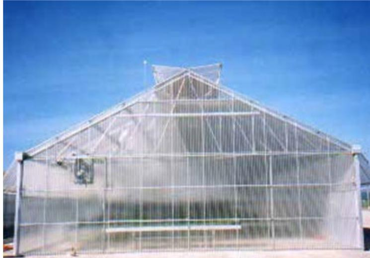
**Figure 3.6** Glass or rigid plastic cladding, used in temperate climates
