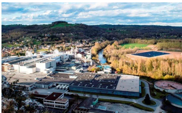
Figure 18 : Photo of the industrial site where the 4,000 m 2 solar thermal field was installed (source: NewHeat)
