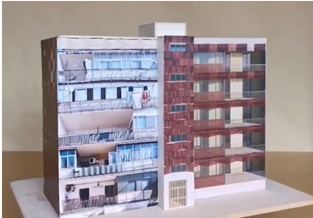
Figure 8a: G1 solution_perforated aluminum panels
