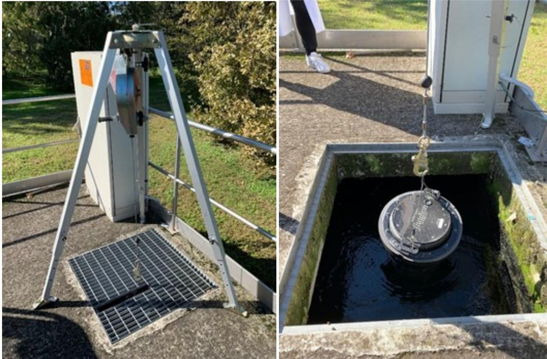
Figure 33: installation of the ALERT System at Peschiera-Borromeo WWTP
