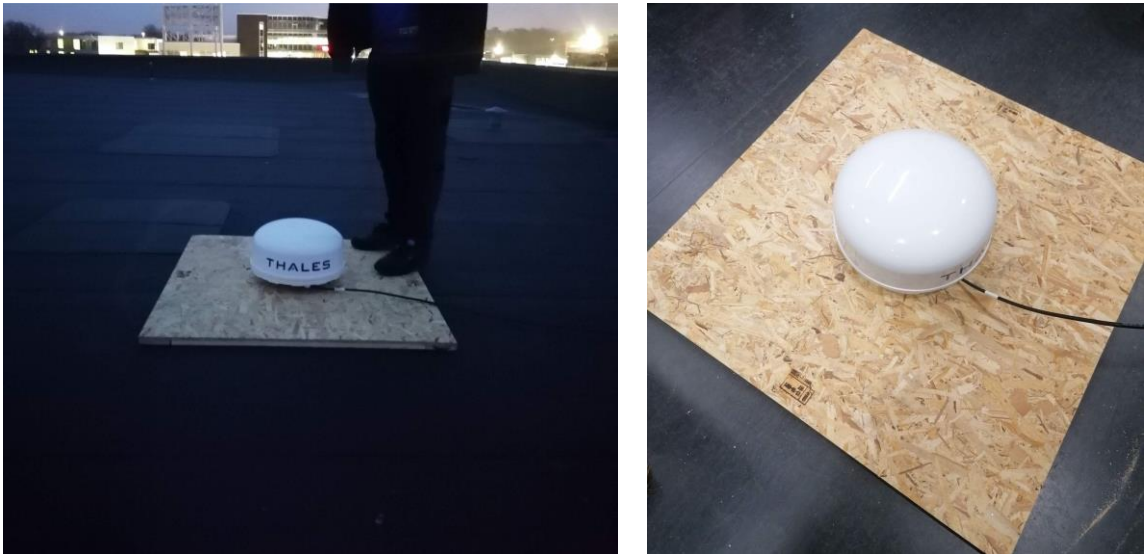
Figure 36. Thales VesseLINK test setup
