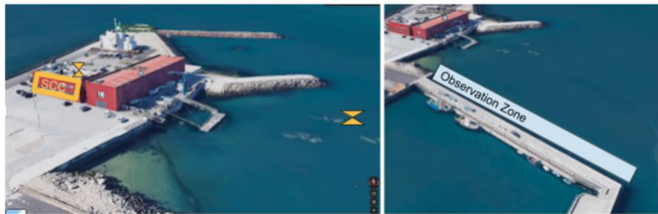
Figure 3. Supervisory Control Centre, observation zone and coastal testbed geography
