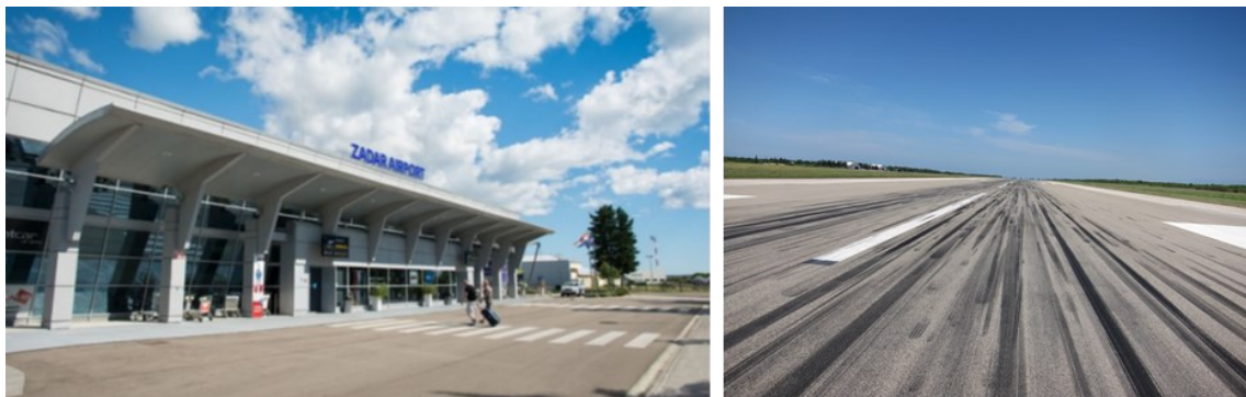
Figure 5.3: Zadar airport terminal building (left) and runway (right)
