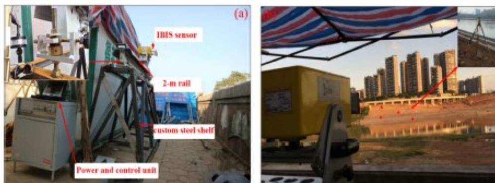
Figure 2.230. Analysis of Baishazhou Yangtze River Bridge using Ground-Based SAR and RAR (Hu et al. 2019).
