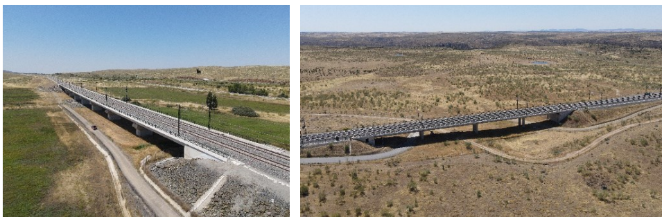
Figure 5.2: Valdelinares Viaduct (left) and La Plata Viaduct (right)
