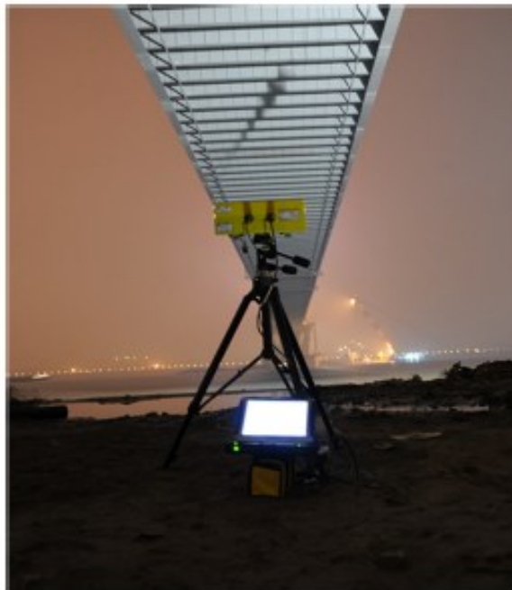
Figure 2.32. Analysis of a steel bridge crossing the Yangtze river in Wuhan, China (Xing et al. 2020)
