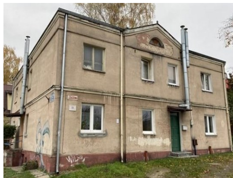
Figure 5.3 Gdynia. Residential Building
