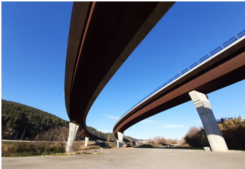
Figure 5.4: Road bridge. Barcelona Area
