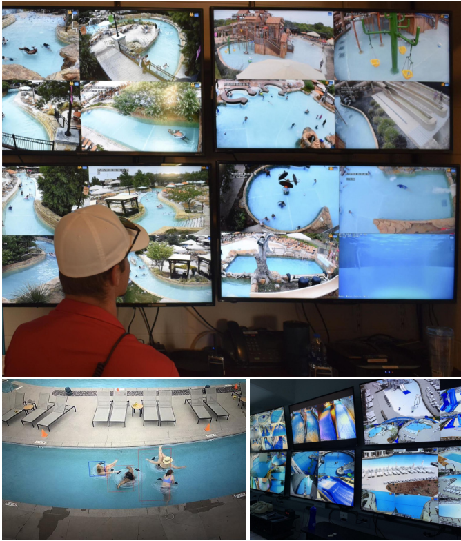
Figure 23. Ellis Aquatic Vigilance System (EAVS) integrates analytics, artificial intelligence and end-to-end monitoring under and above water and on land to elevate swimmer safety, drowning prevention and security [25].
