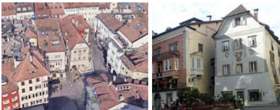
Figure 13: Principal facade on Kornplatz, Waaghaus. Source http://www.3encult.eu/en/project/welcome/PublishingImages/Waaghaus%20copy.jpg
