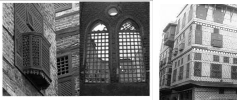
Figure 25: Left: the used screens (Mashrabiya), right: a building facade with small openings 7 .
