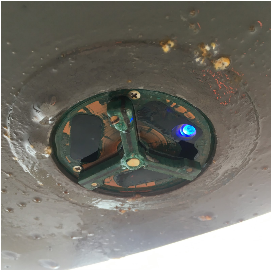
Figure 15. ADCP installed on a Sairdrone vehicle.
