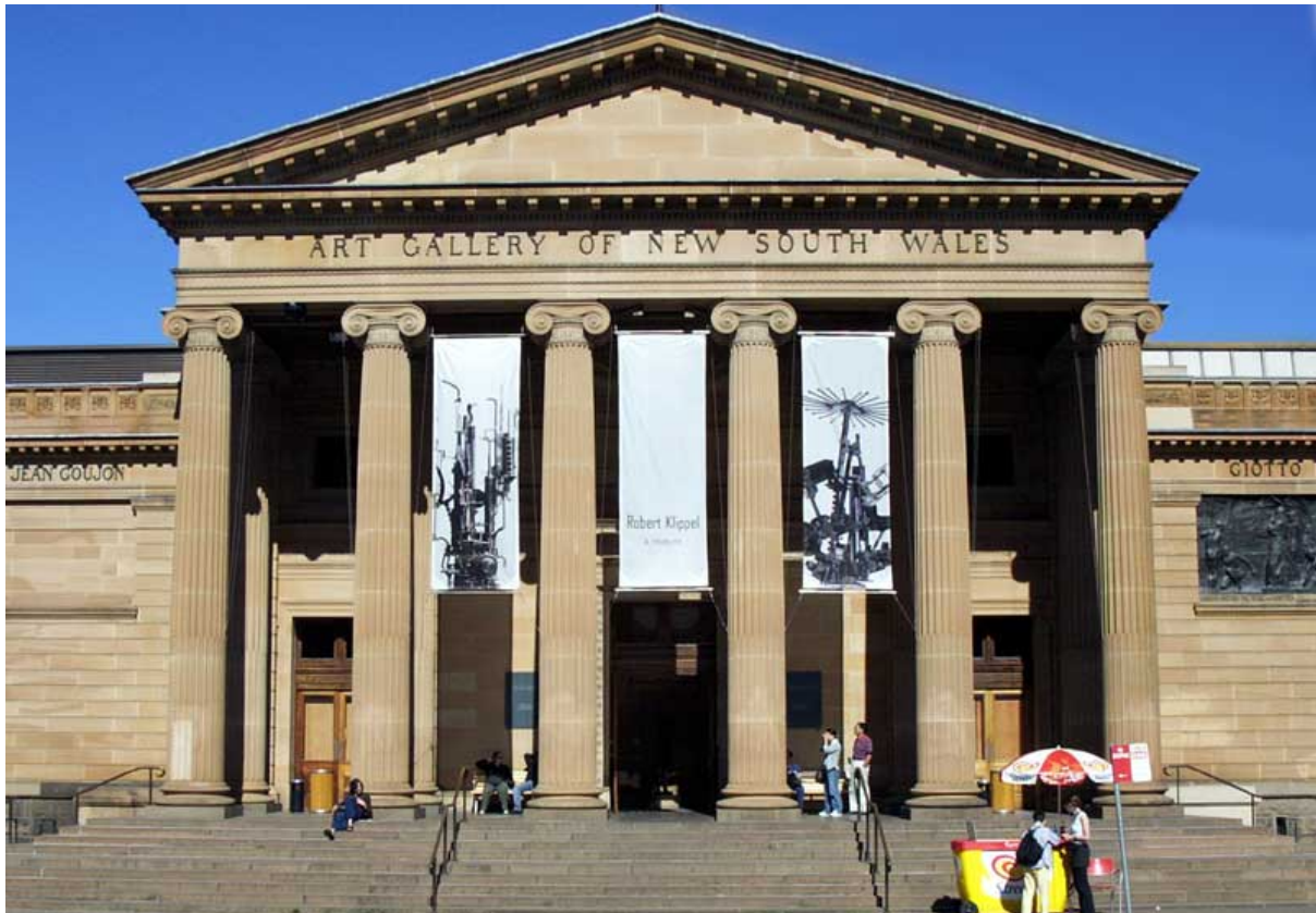
Figure 1. The façade of the Art Gallery of New South Wales.
