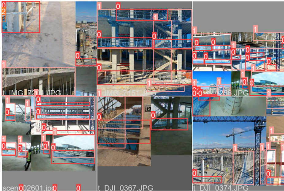
Figure 2: Tiled image samples (3 x 2 tiling) of the augmented data with artificial scaling, shearing, flipping and mosaic of the original dataset images.
