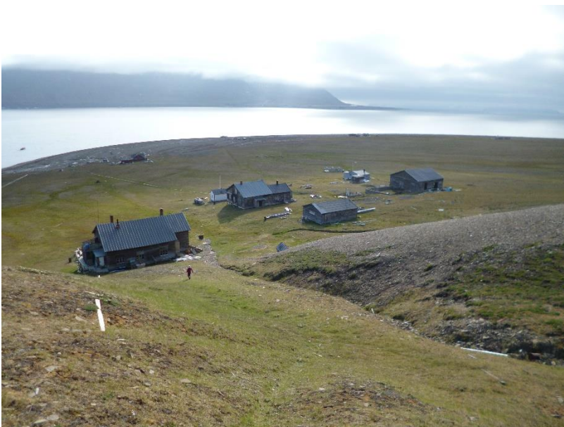
Fig. 2. Reconnaissance at Hiorthhamn. These are some of the original buildings from Advent City. Photo: Frigga Kruse, 2014.
