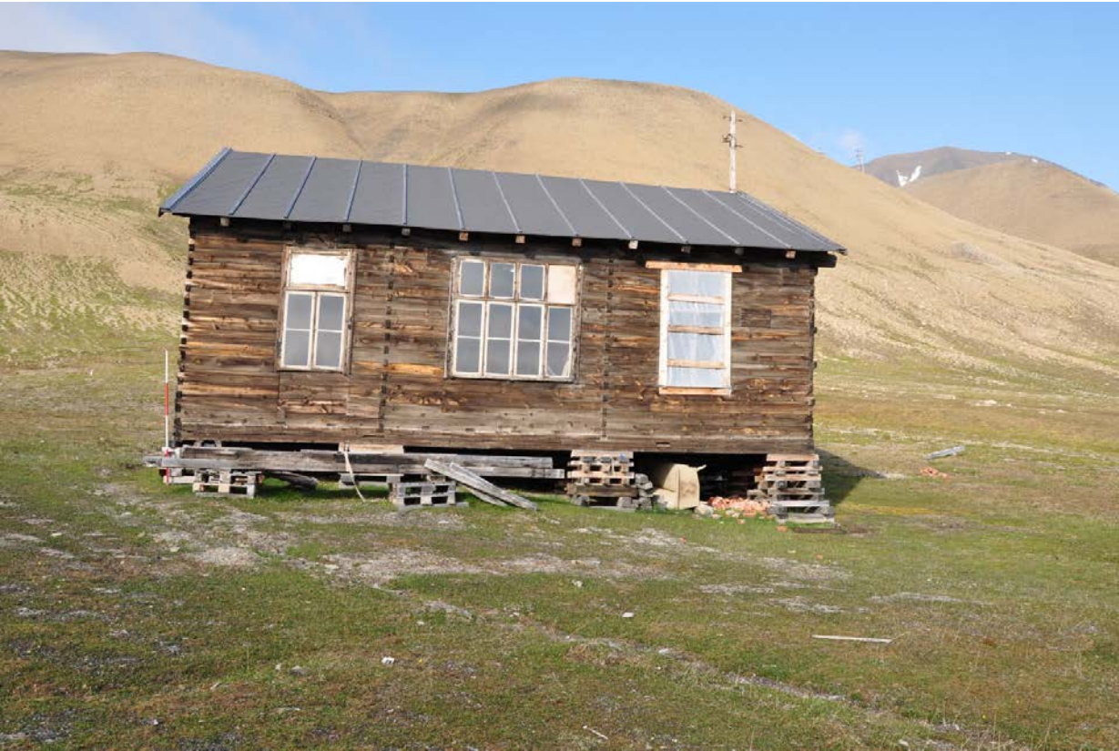
(8) Building G (living quarters) in Hiorthhamn, scale 2m, looking NE. (Photo: S. Dresscher, 2014.)
