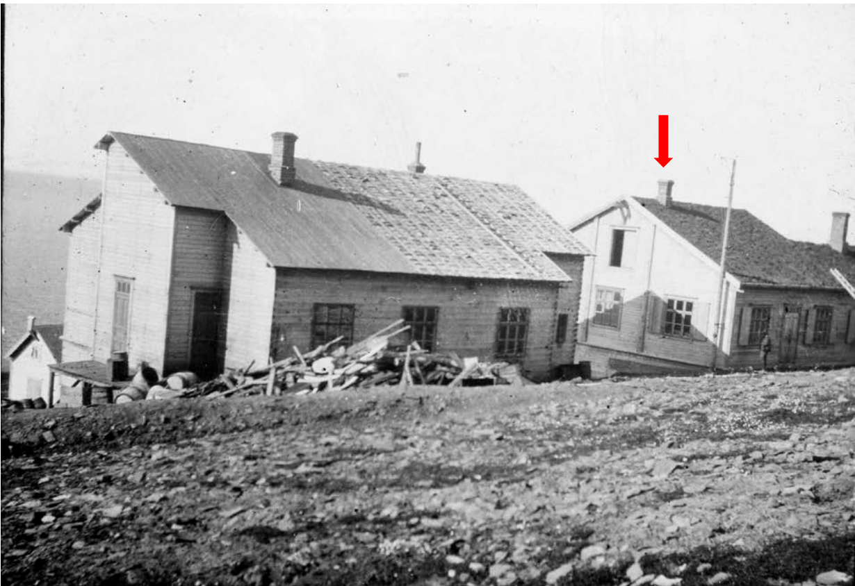
Building C originally stood in Advent City, but its former function is not known, looking W. (Source unknown.)
