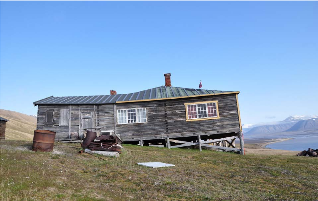
(5) Building F (administration building including telegraph facility) in Hiorthhamn, scale 2m, looking SE. (Photo: S. Dresscher, 2014.)
