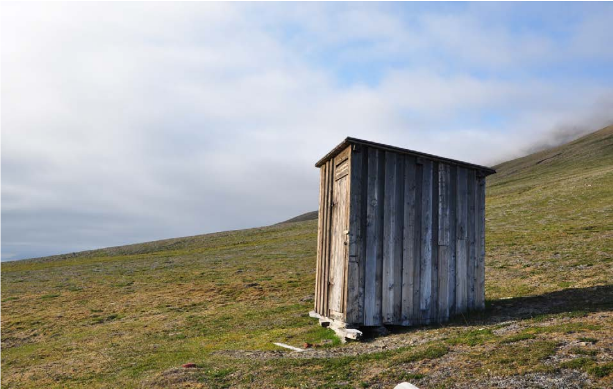
(10) This is an outhouse to the north of building G in Hiorthhamn, looking NW. (Photo: S. Dresscher, 2014.)
