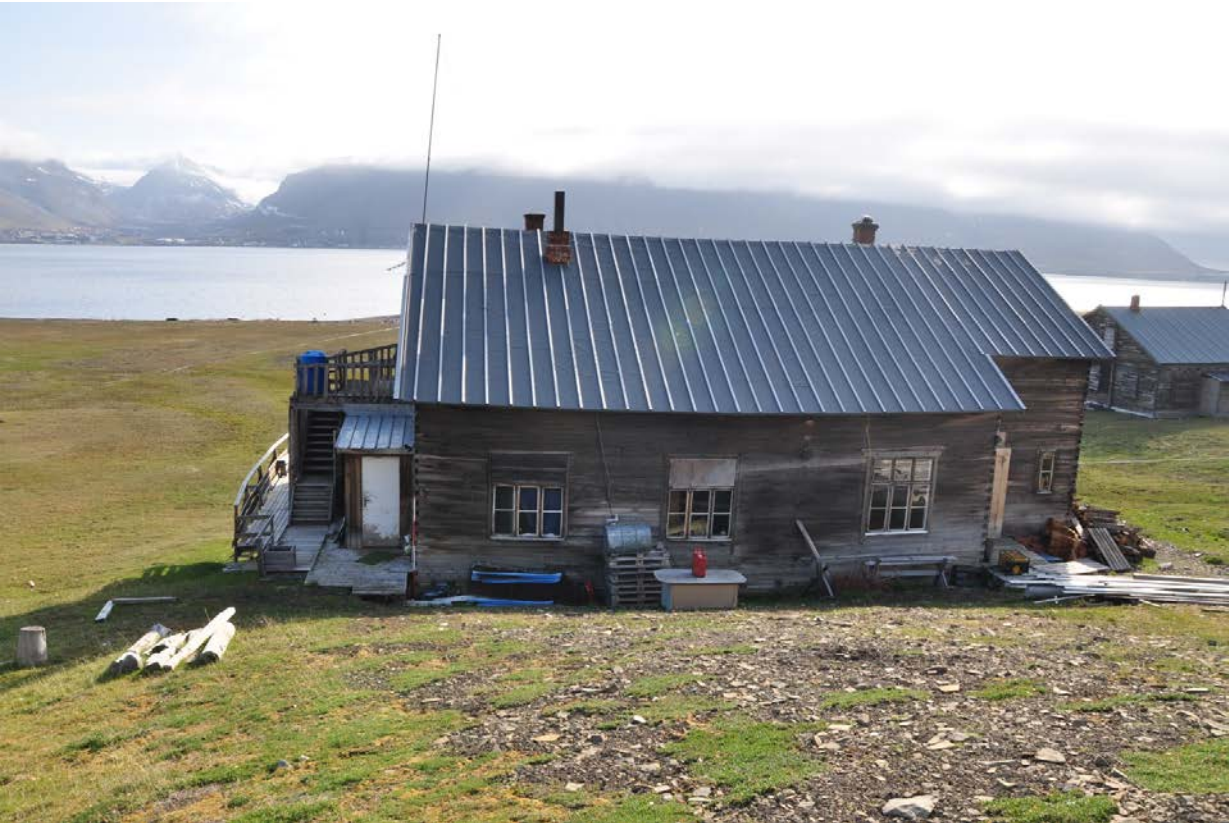
(2) Building E (large mess hall, bakery) in Hiorthhamn, scale 2m, looking SW. (Photo: S. Dresscher, 2014.)
