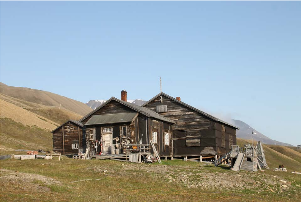
(12) Building C (living quarters) in Hiorthhamn, looking E. (Photo: S. Dresscher, 2014.)
