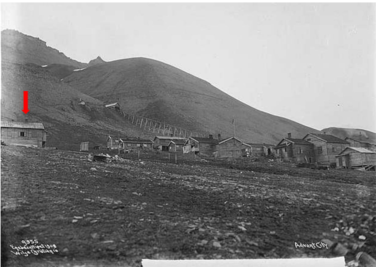
Building G used to stand in Advent City, where it probably had the function of a club house, looking E. (Source: Norsk Folkemuseum, NF.W 09355.)
