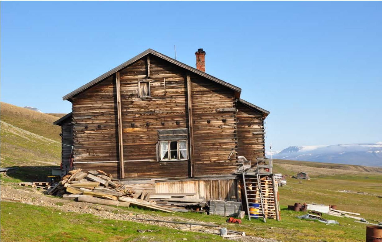
(3) Building E (large mess hall, bakery) in Hiorthhamn, scale 2m, looking SE. (Photo: S. Dresscher, 2014.)
