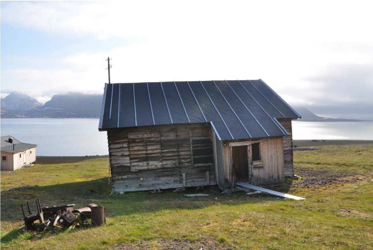
(10) Building G (living quarters) in Hiorthhamn, scale 2m, looking SW. (Photo: S. Dresscher, 2014.)
