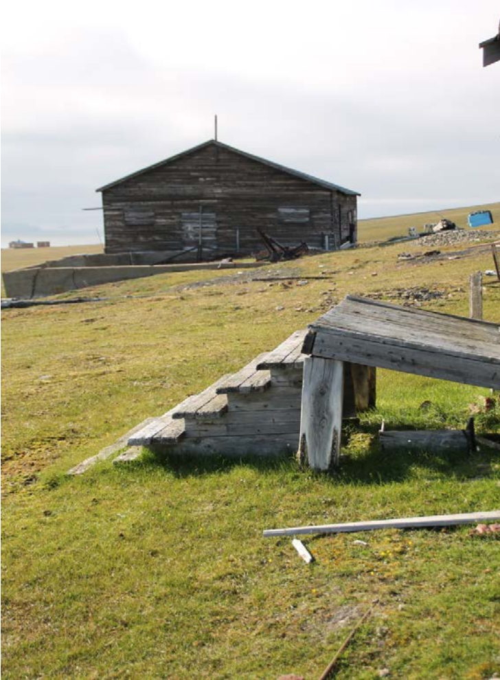
(6) Building A (storage facility, machine shop) in Hiorthhamn, looking NW. (Photo: S. Dresscher, 2014.)
