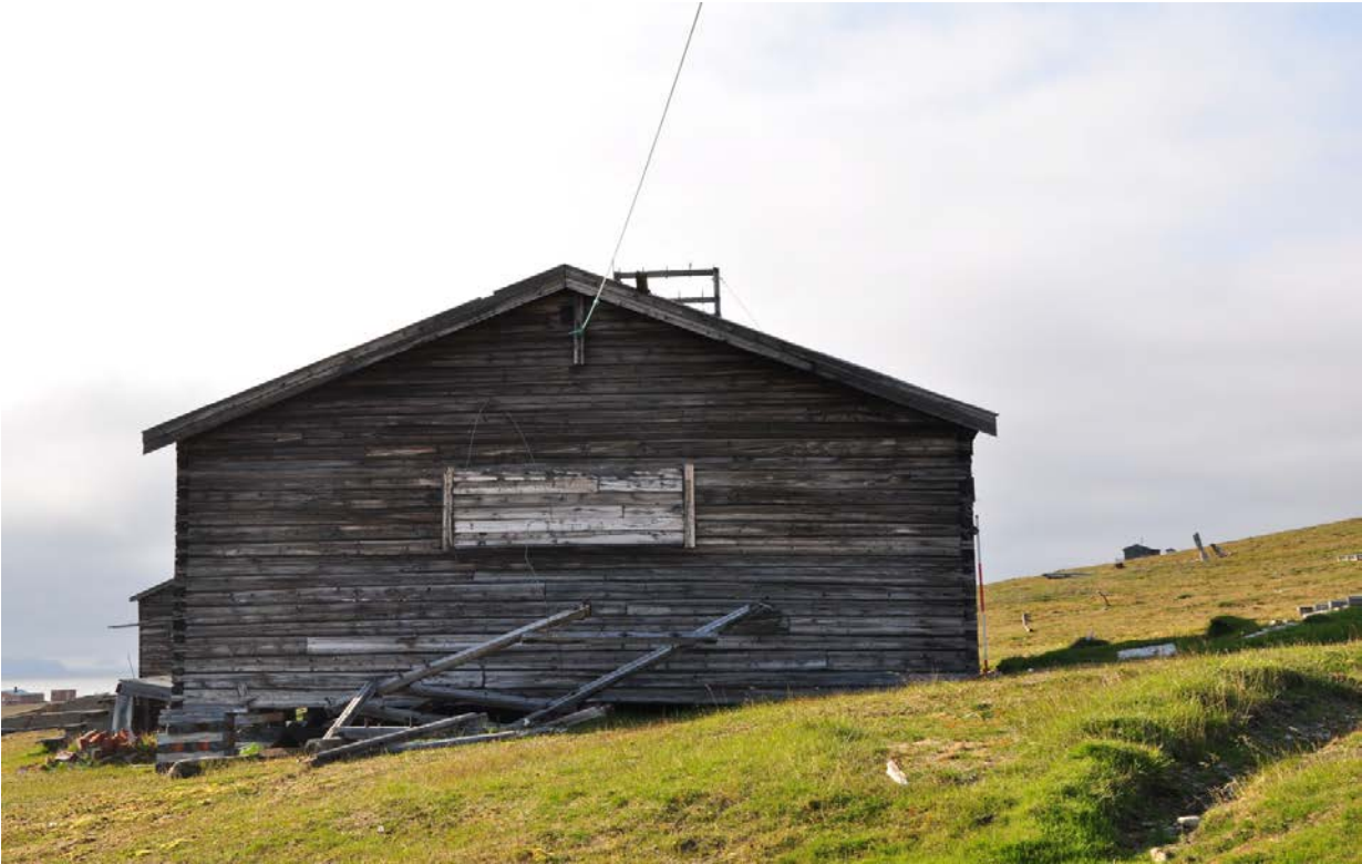
(7) Building B (telegraph, general store and provision storage) in Hiorthhamn, scale 2m, looking NW. (Photo: S. Dresscher, 2014.)
