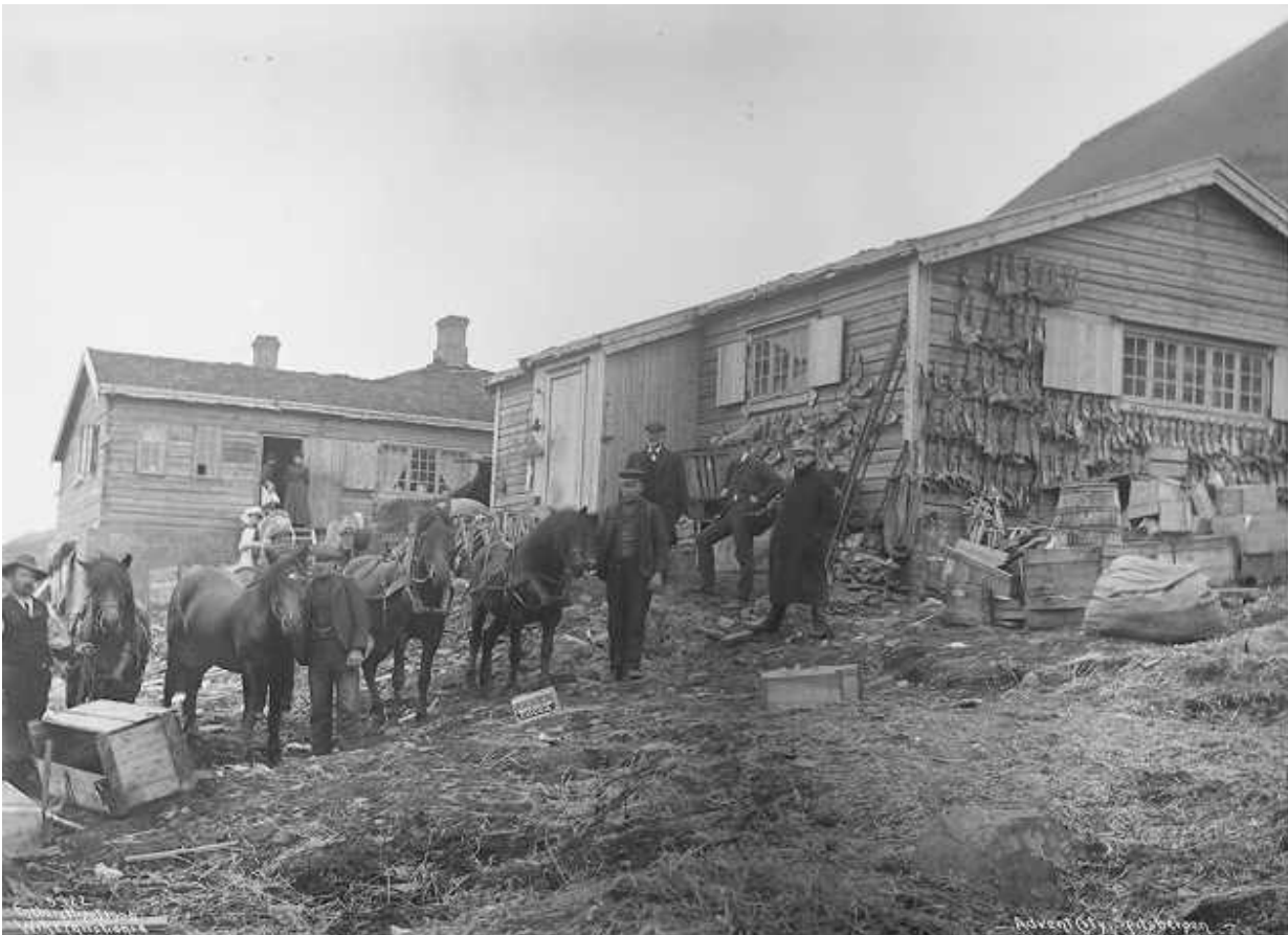
Building B originally stood in Advent City and probably had the same function of being provision storage, looking N. (Source: Norsk Folkemuseum, NF.W 05522.)
