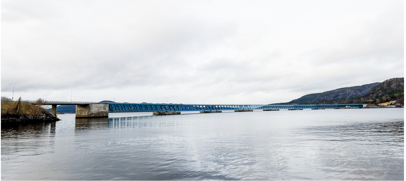
Figure 1. Photograph of the Bergsøysund Bridge. Photo: NTNU/K.A. Kvåle.
